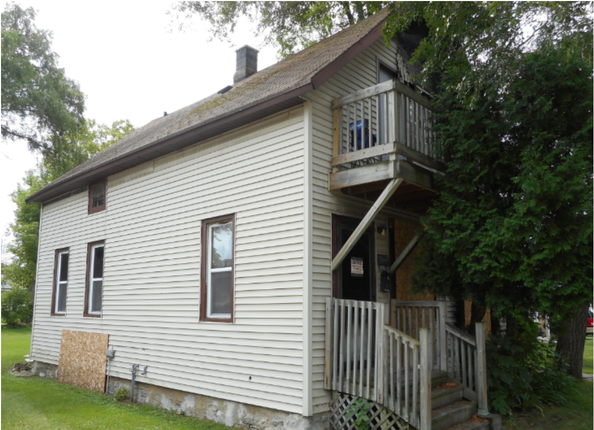
143 Cleveland Street (Raze or Remove – repairs would exceed 50% of assessed value)
