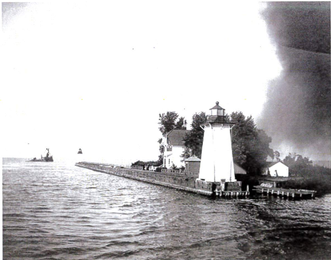
Original site of the range lights with support building.
