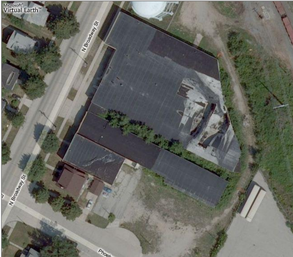
Aerial view of collapsing warehouses, 2007.
