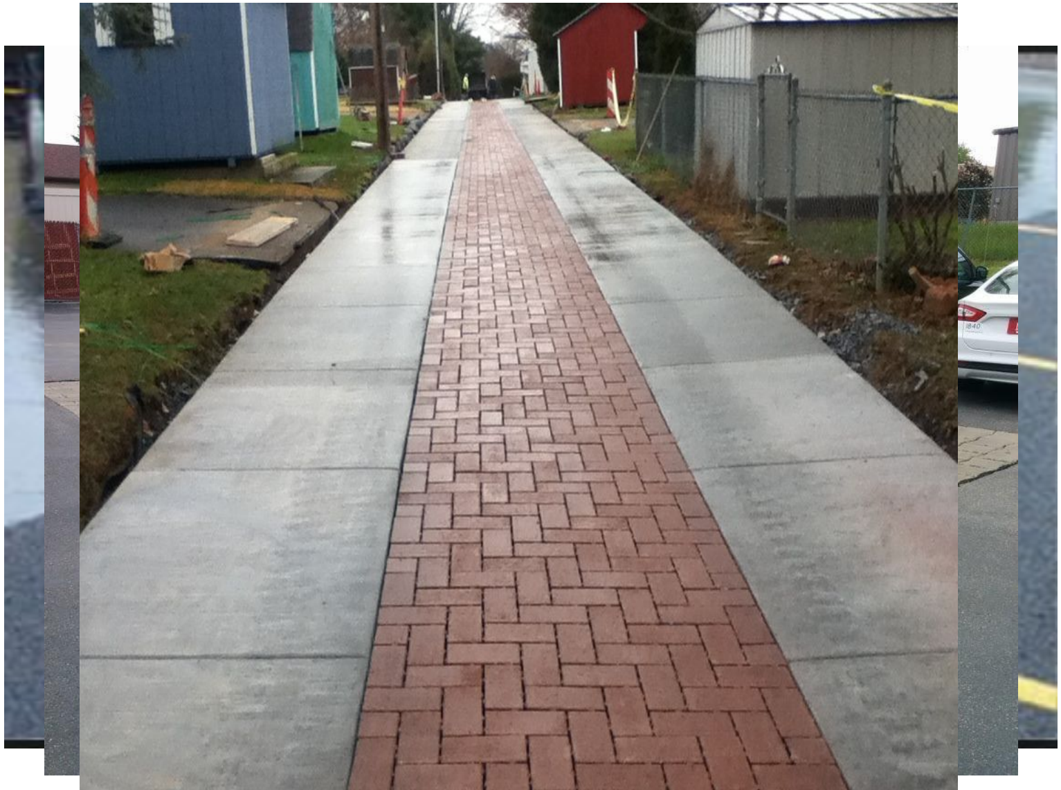
Permeable Pavements and Pavers
