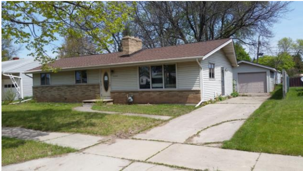
(Existing structures to be demolished.)
