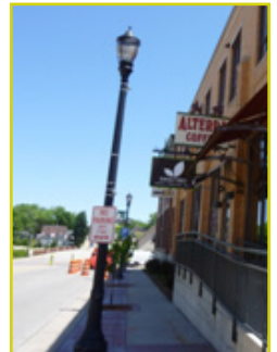
ABOVE: Pedestrian-scale traditional pedestal lighting.
