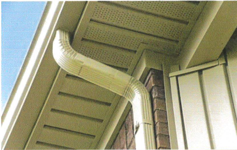
Pictures of soffit, fascia, and gutters from the Creative Homes Technology website
