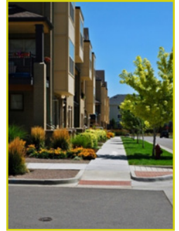
ABOVE: Sidewalks with terraced areas for areas off main roads.
