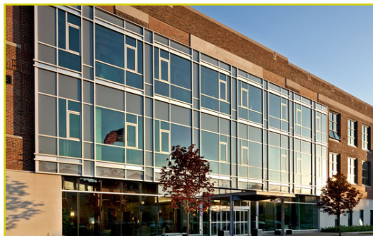
RIGHT: Example of a quality building design that incorporates quality materials
