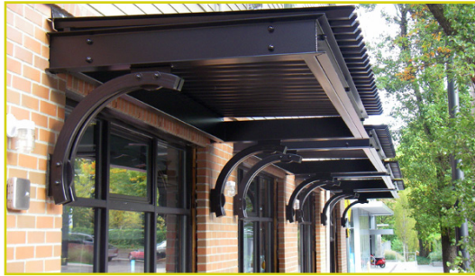
LEFT: Example of building awnings
