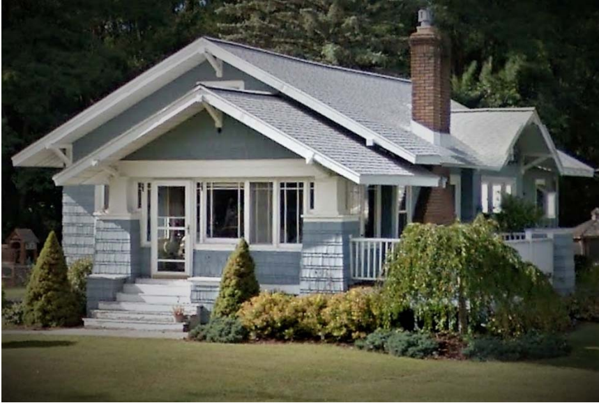
(tastefully enclosed porch & side deck)
