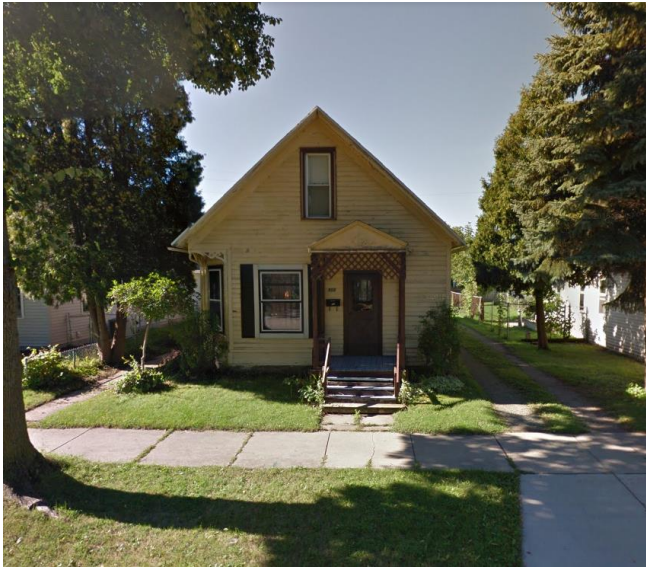
Previous structure - demolished Summer 2019
