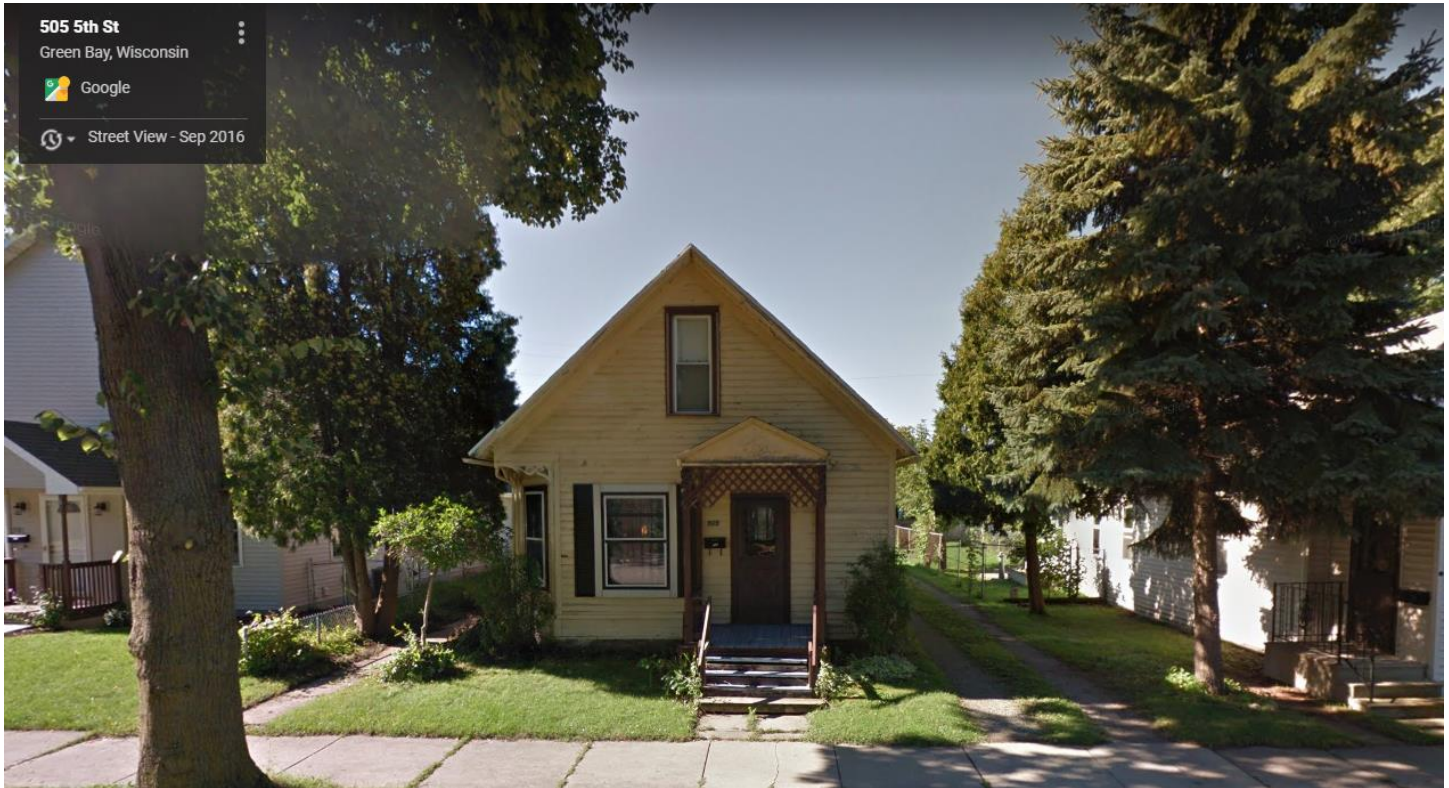
Street view of 505 5 th Street, Prior to Demolition
