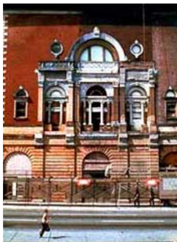
Ninety years of accumulated dirt and pollutants are being removed from this historic theater using an appropriate chemical cleaner, applied in stages. Photo: Richard Wagner, AIA.
