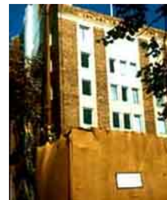
The lower floors of this historic brick and architectural terra-cotta building have been covered during chemical cleaning to protect pedestrians and vehicular traffic from potentially harmful overspray. Photo: NPS files.
