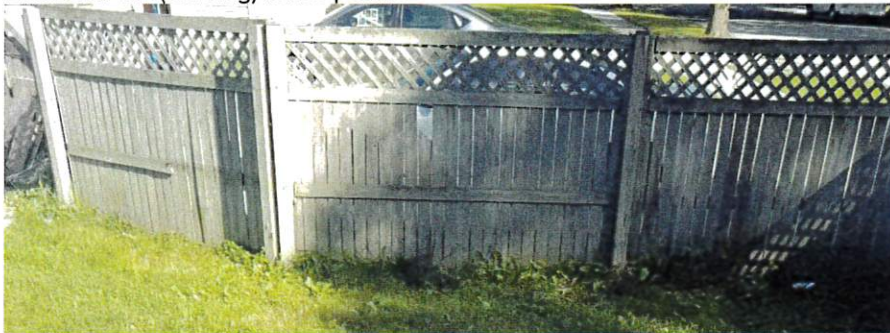
Photos of old (existing) fence panels
