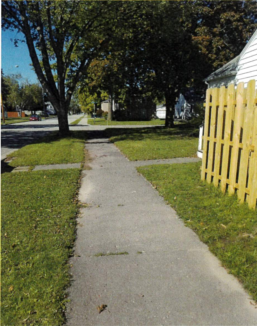
2. From driveway looking towards Winford Av
