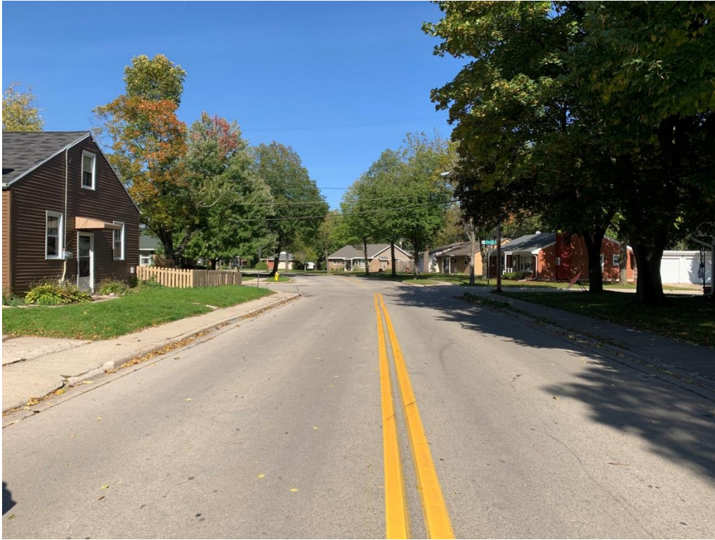
Figure 3a – Northbound Gross Ave approaching St Paul St (near count location)
