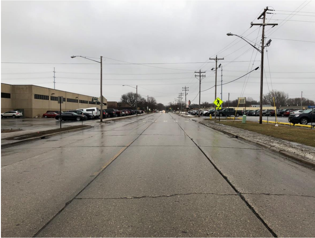
Figure 4 – Eastbound Radisson St at Green Bay Packaging Midblock Crosswalk
