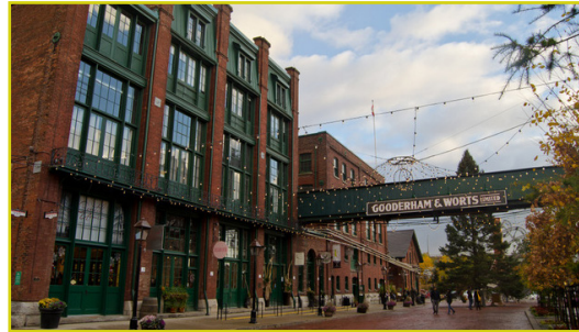
LEFT: Example of urban, industrial-themed buildings and district and zero lot line development and proper window transparency
