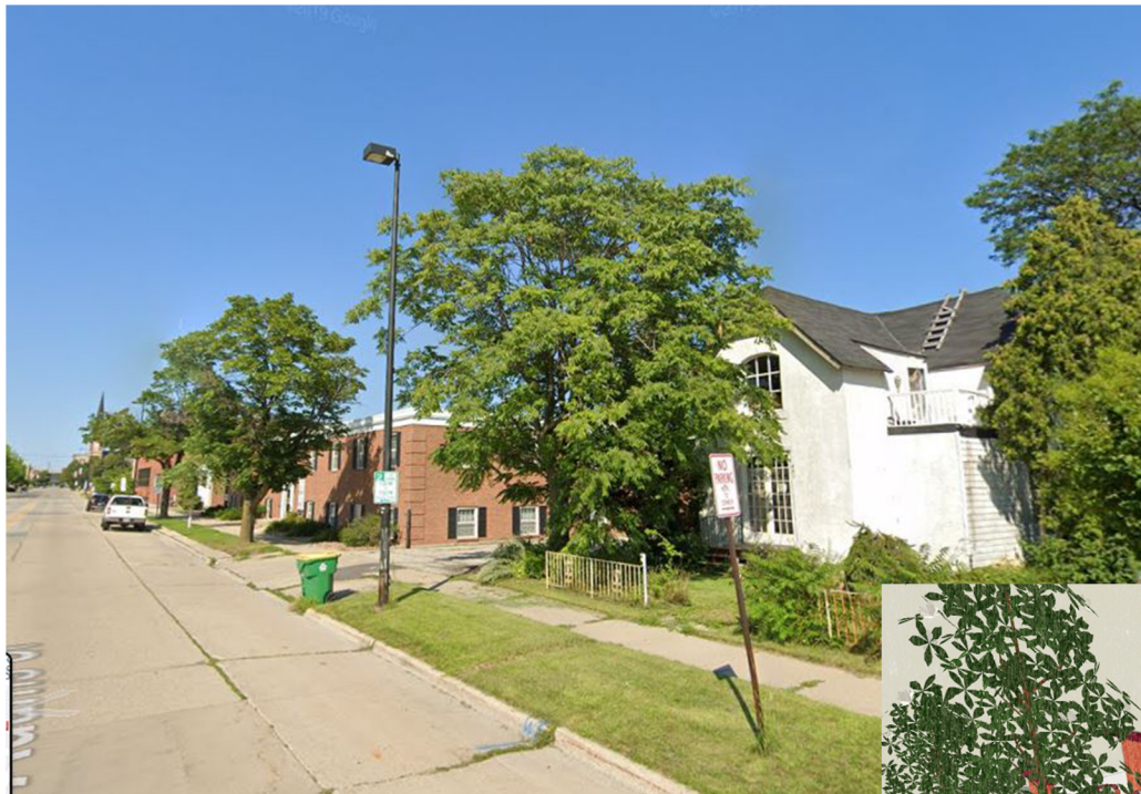
Previous/Existing Condition (adjacent condemned home)
