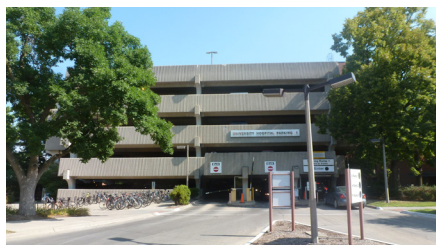
University of Iowa Hospital Parking Ramp (HR1)
