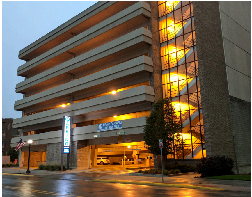
River's Landing Parking Ramp on Douglas Street
