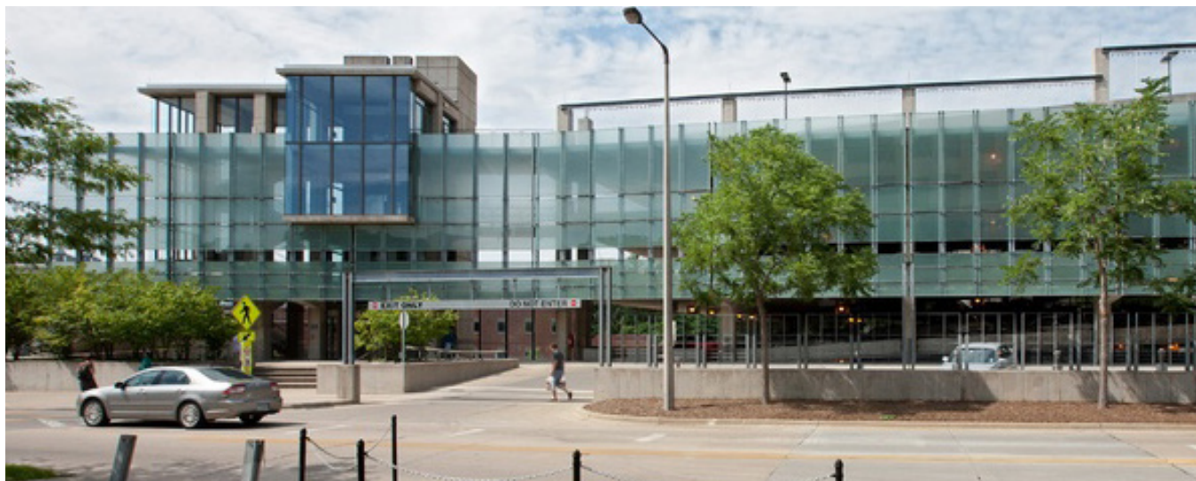
Newton Road Ramp (NR)
