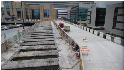
Repairs phased to maintain traffic flow
