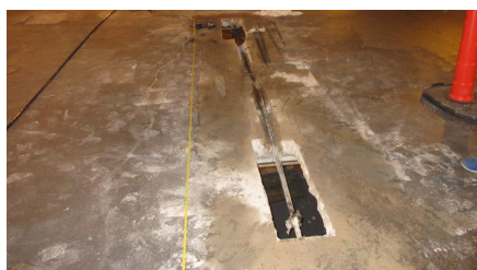
A button-head tendon repair in progress, which included cutting out the corrosion damaged section of the tendon, adding a tendon coupler, a new tendon, and a stressing-coupler that allowed the tendon to be restressed to the calculated force
