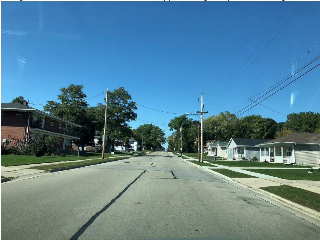
Figure 3b – Westbound Western Ave approaching Maryhill Dr looking West
