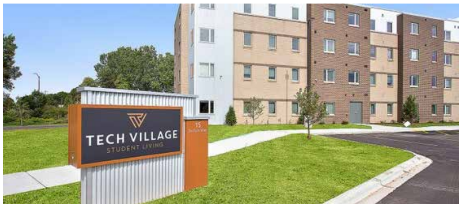
Northeast Wisconsin Technical College Housing
