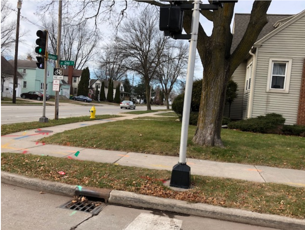
Figure 4I – Southbound Gray St at Dousman St looking West (Right)
