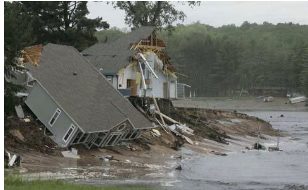
Figure 15: Lake Delton, WI Dam Failure Flood Damage Source: Twincities.com
