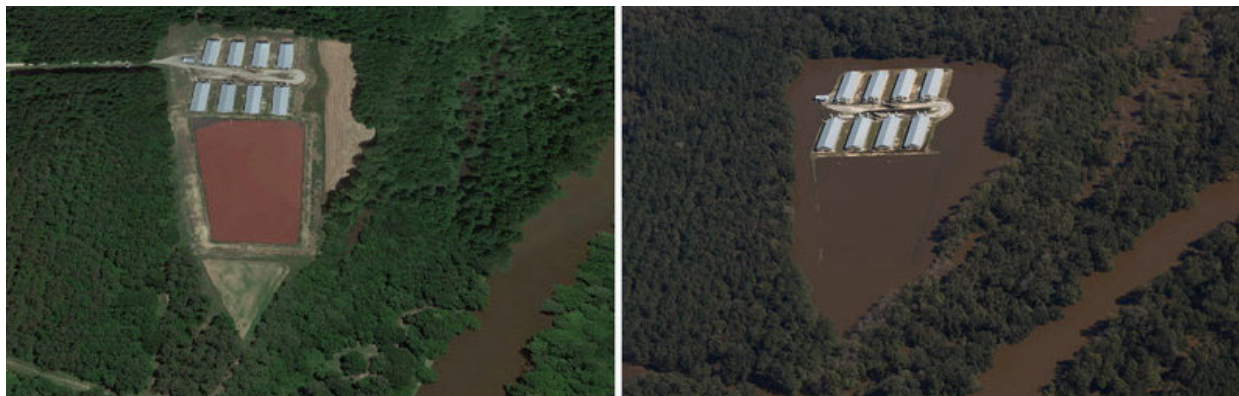
Figure 1: Manure pit/lagoon near a river before and after flooding event. Source: NPR
