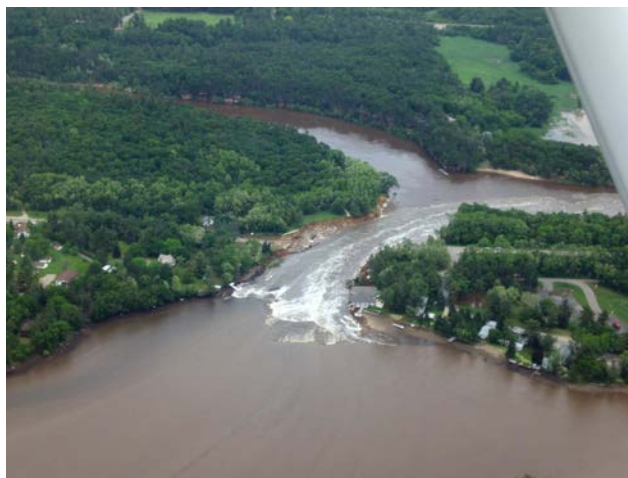
Figure 14: Lake Delton Dam Failure Source: wiscnews.com
