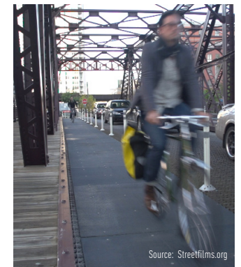
Bike Lane on Lift Bridge in Chicago, IL
