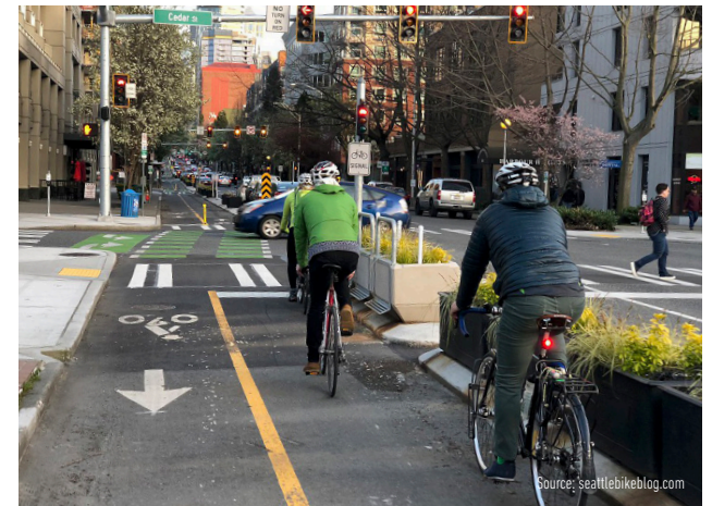
Planter Buffer along Two-way Bike Lanes in Seattle, WA
