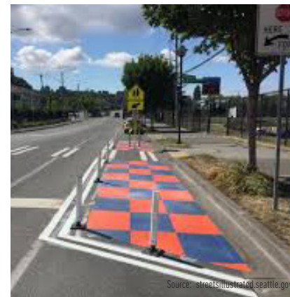
Painted Curb Extension in Seattle, WA
