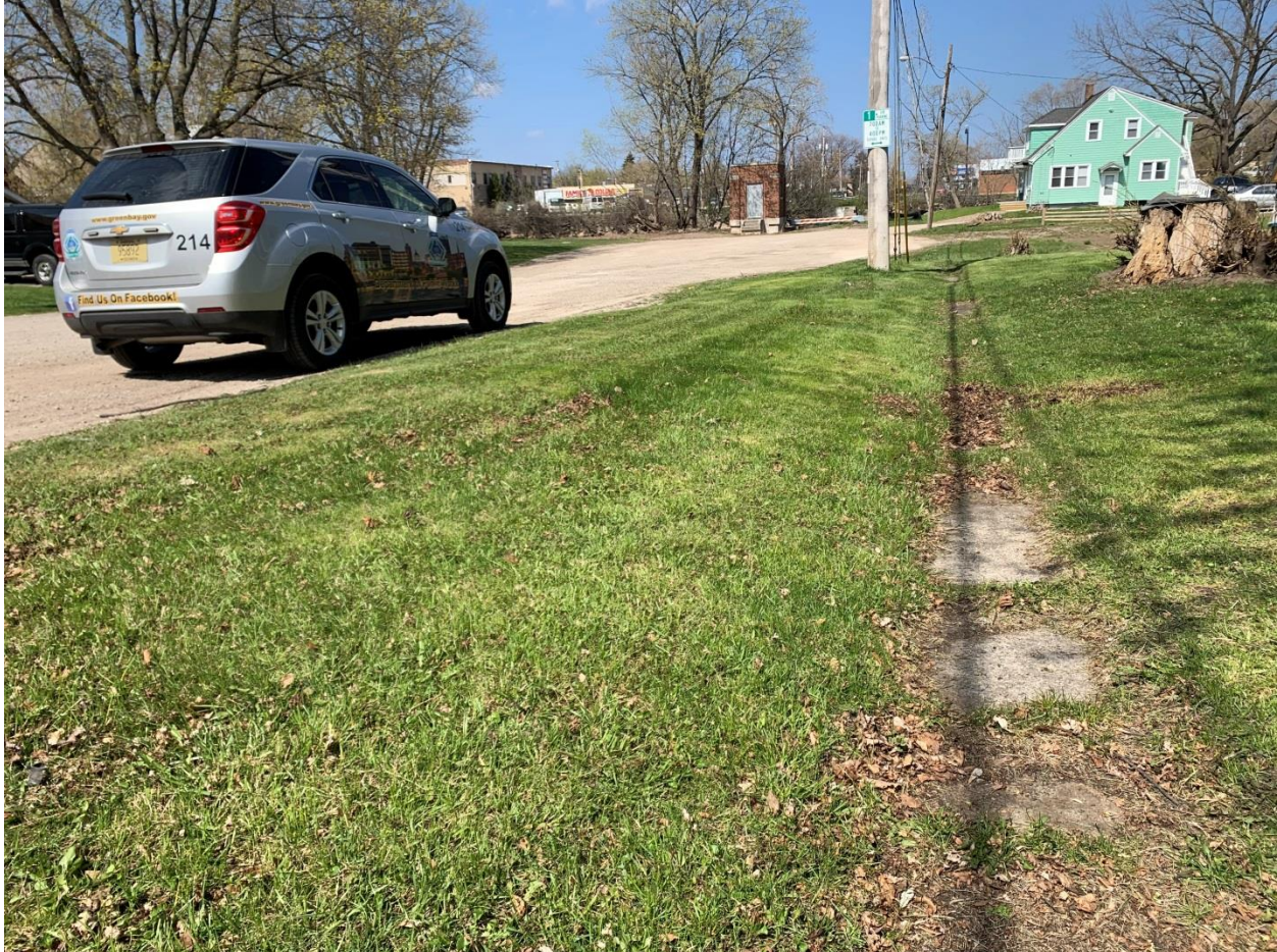
Figure 2 – Existing Sidewalk, east side of N Irwin Ave
