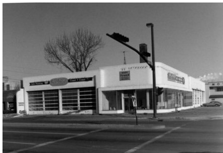
Earl Schieb Auto Painting Photo of Property
