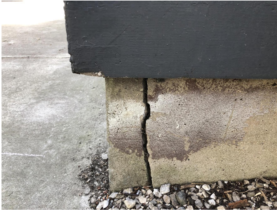
Garage Floor Cracks - (tripping hazard)
