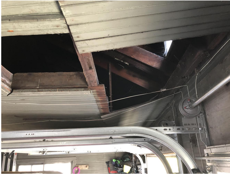
Ceiling Rafters (shown above ceiling where fasteners are failing)
