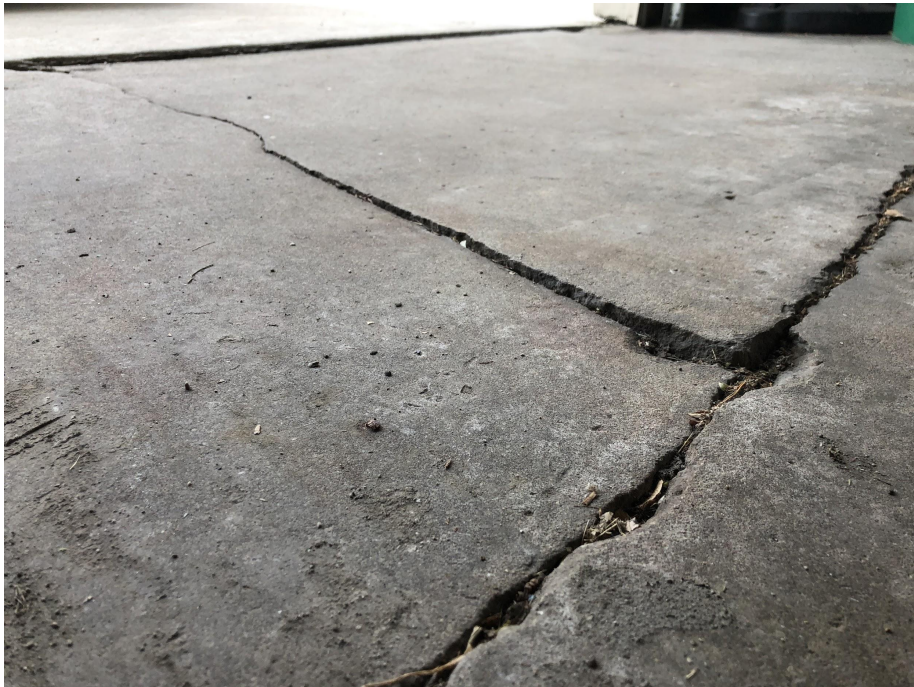
Garage Floor Cracks - (tripping hazard)
