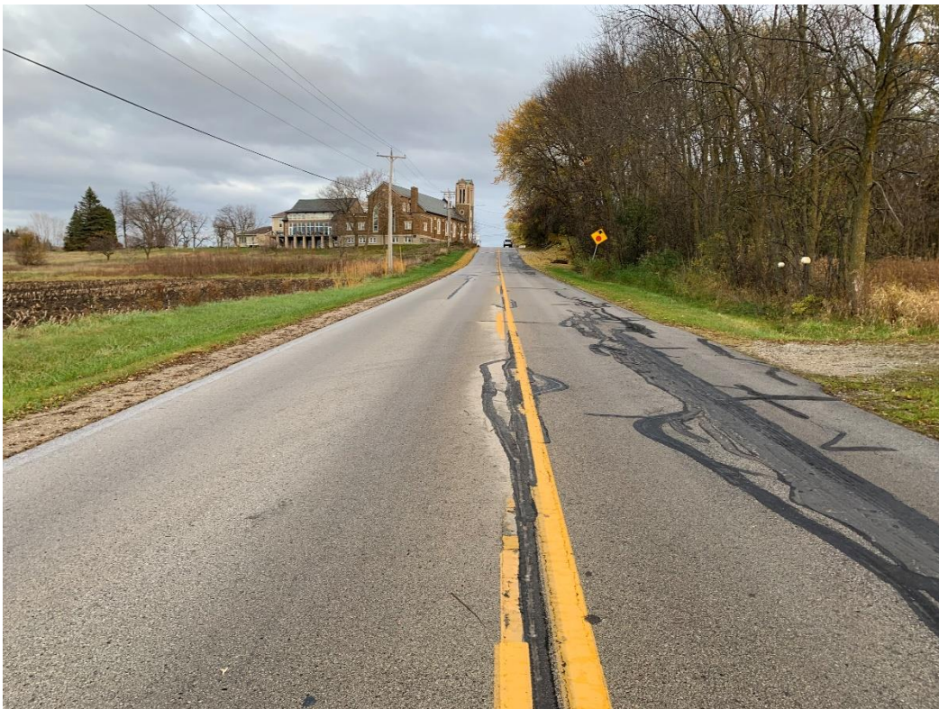
Figure 3a – Eastbound Church Rd from Sussex Rd to Bay Settlement Rd (near count location)
