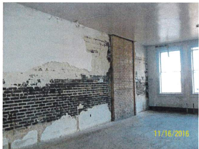
3 rd floor plaster on north bearing wall
