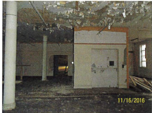
2 nd floor columns and elevator shaft
