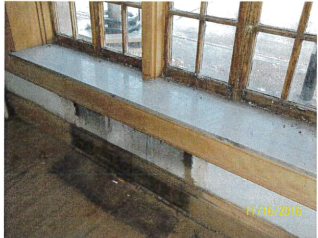
Marble sill at east windows
