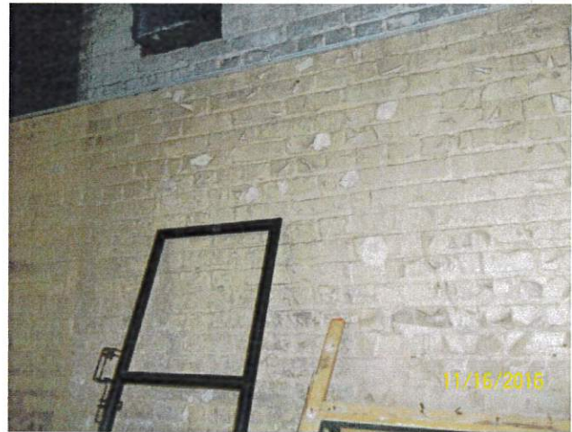
Basement bearing wall
