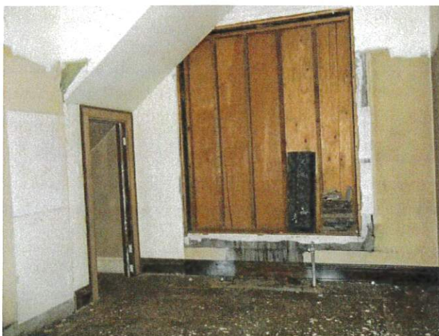
Removed window toward alley
