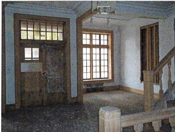
Entry, former office, and stripped stair rails
