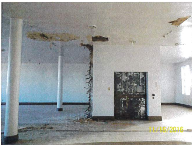
3 rd floor columns and elevator shaft
