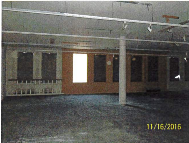
2 nd floor column
