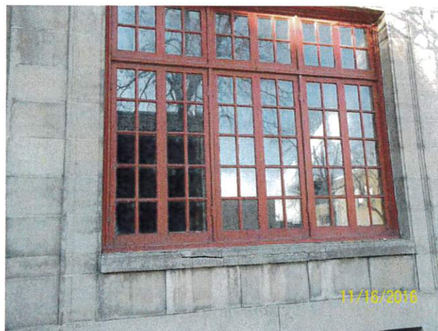
Cracked sill
