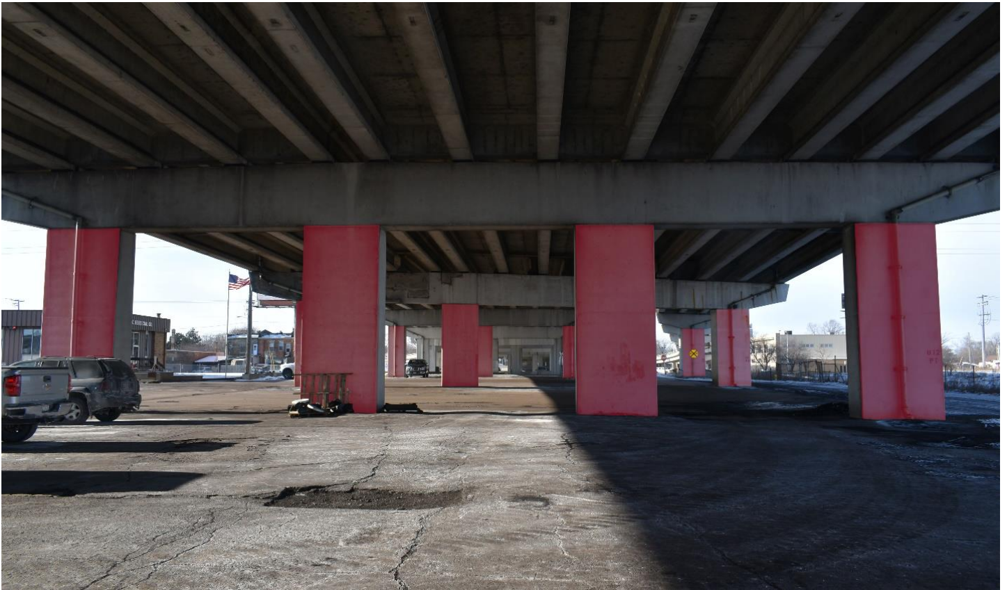
View looking west. Pillar rows #4 – #6 highlighted. City of Green Bay photo.
