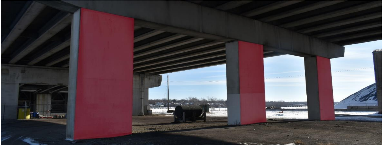
Highlighted areas in red indicate potential areas of focus. Row #1 closest to the river looking southeast
