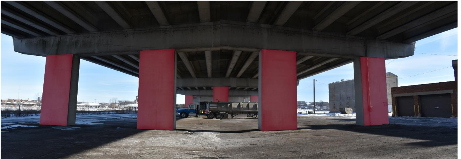
Panorama image compiled to show first two rows of pillars nearest the river's edge. View looking east. City of Green Bay photo.
