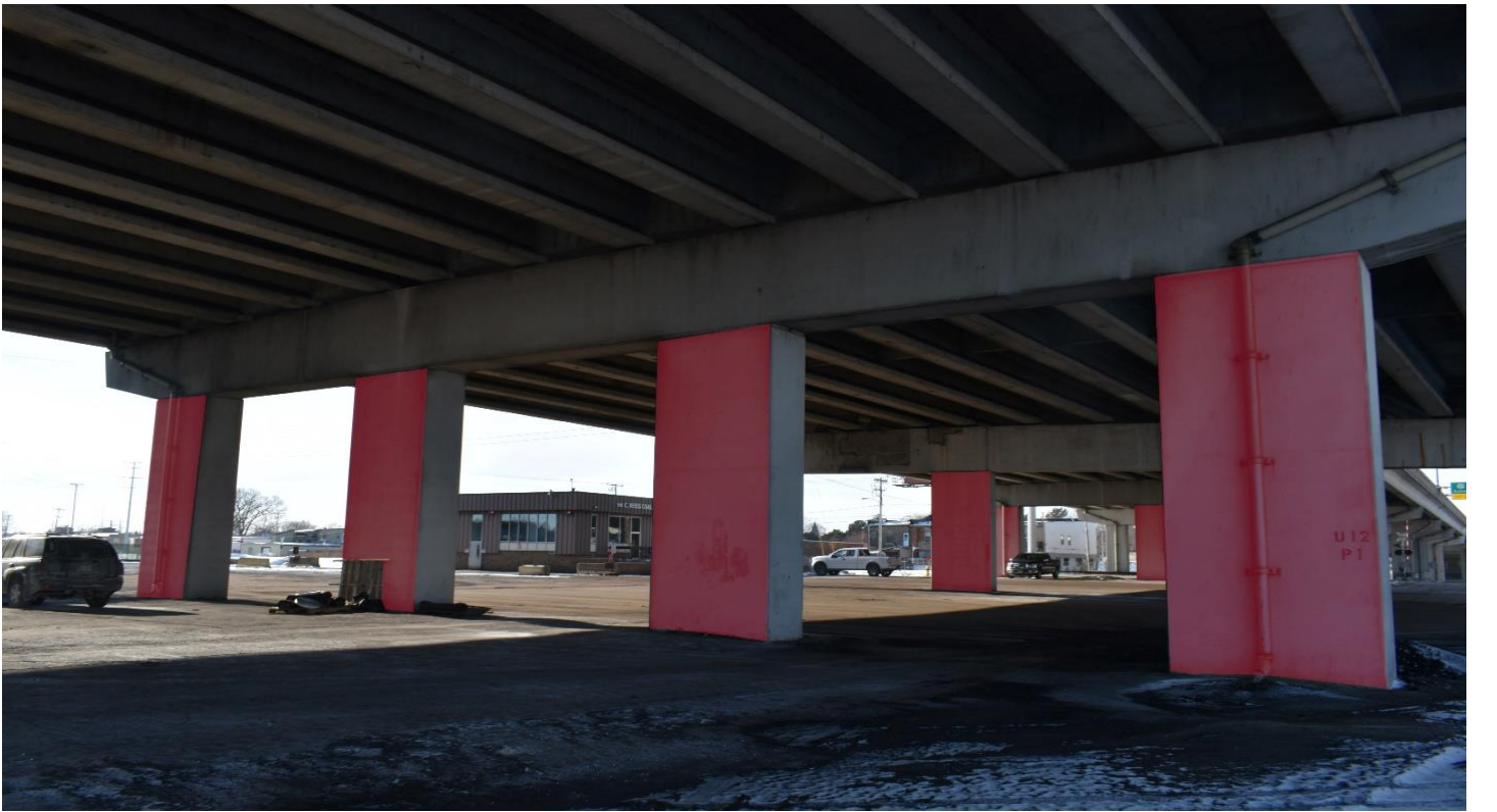
View looking southwest. Pillar row #4 closest in this image. City of Green Bay photo.
