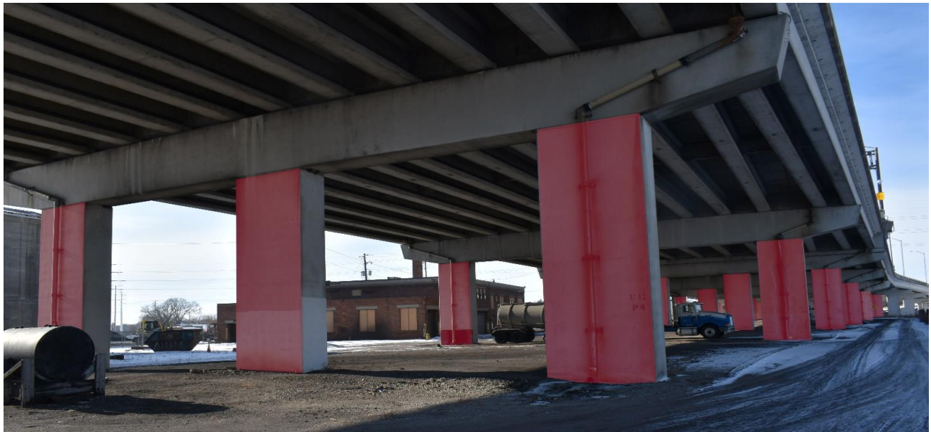
View closest from the river edge looking southwest over the project area of focus – Pillar rows #1 - #6 highlighted. Pillar row #1 closest. City of Green Bay photo.
