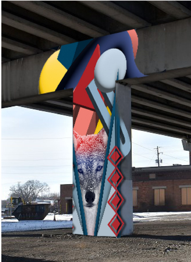
ROW1 CENTER COLUMN LOOKING WEST
