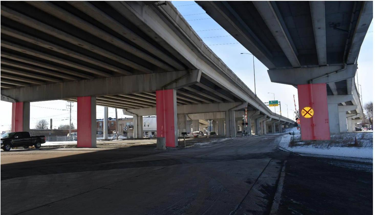
View looking west. Pillar row #6 highlighted. City of Green Bay photo.
