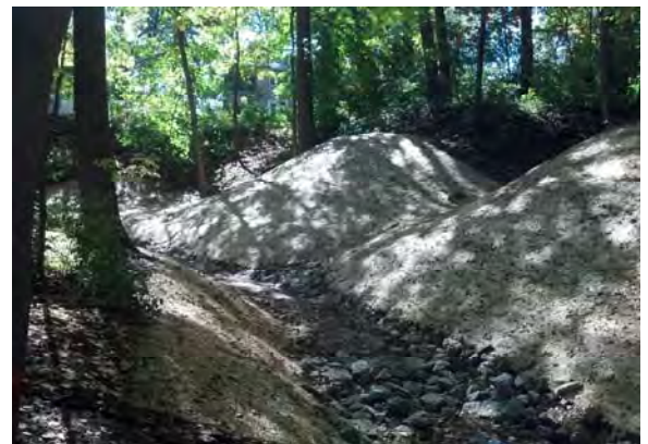
STEEP SLOPE REPAIR
