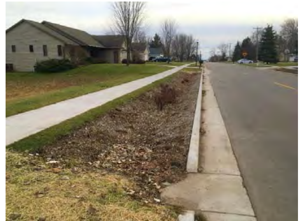
Biofilters located in the terrace
