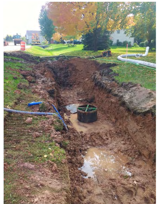
DOUBLE RING INFILTRMETER TESTING
