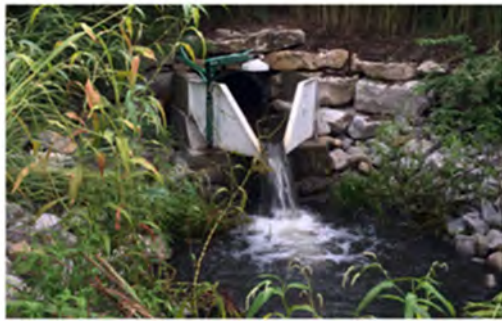
BMP retrofit installed to measure flow
