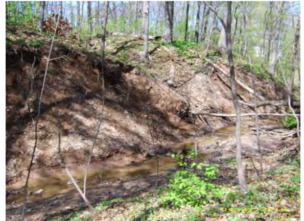
PRE-PROJECT BANK EROSION
