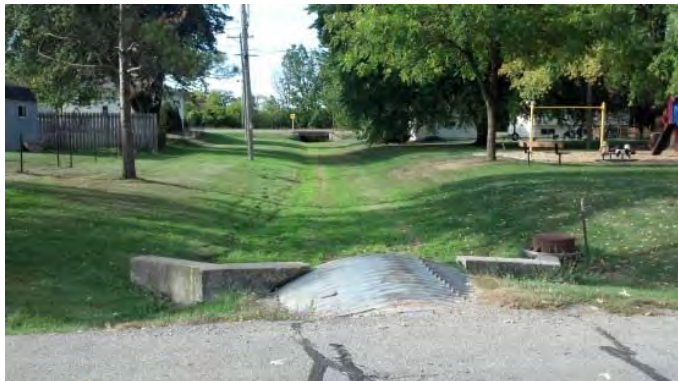
Waterway and culverts
