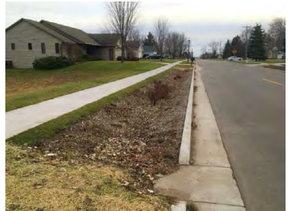
Biofilters located in the terrace
