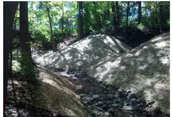
STEEP SLOPE REPAIR
