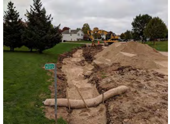
STREET RAIN GARDEN
