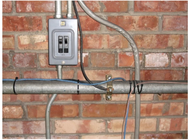
Cable attached to standpipe
