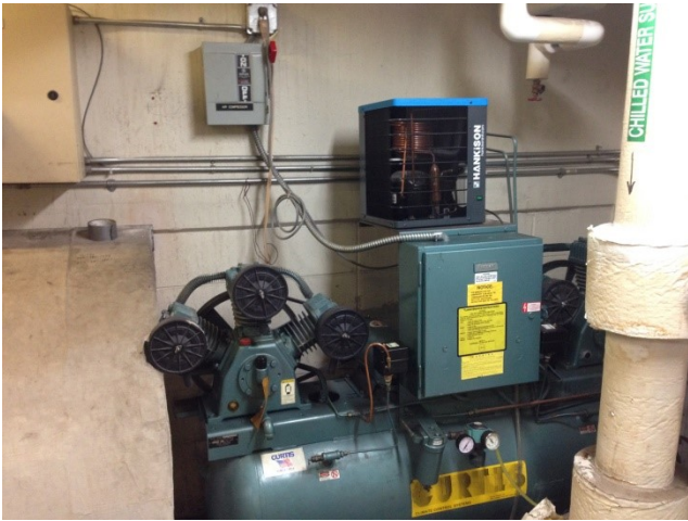
Temperature control air compressor
