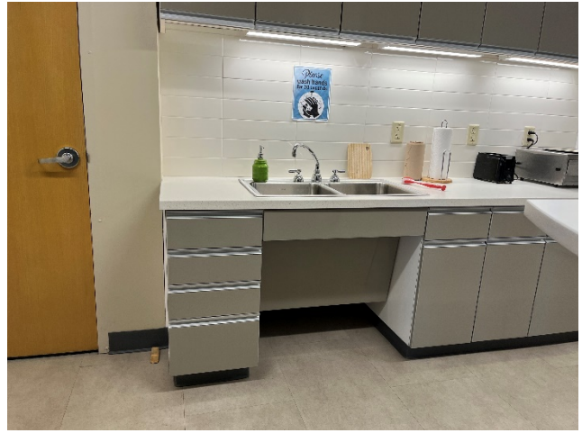
Sink with front-approach accessibility
