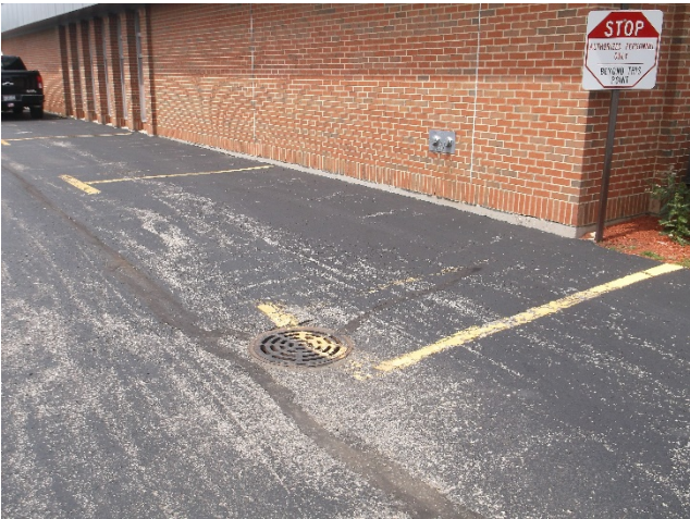
Parking lot- catch basin
