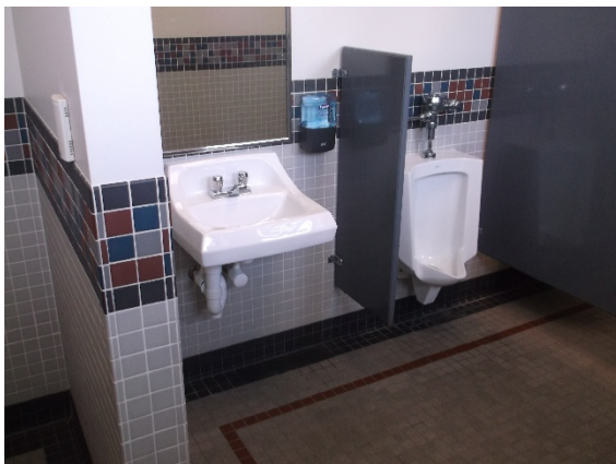
Lavatories – 1 st floor public men's
