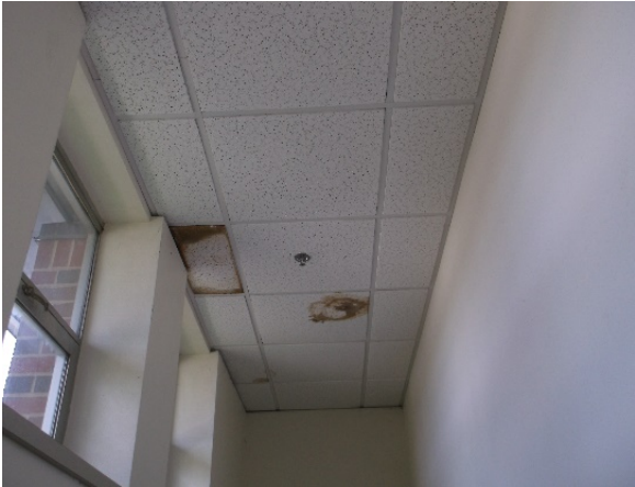
Sprinkler head in stairwell
