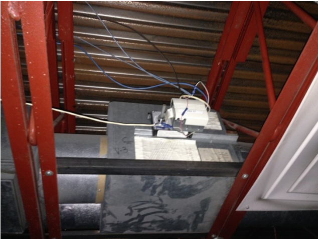
VAV terminal (no reheat)
