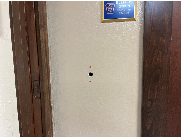
Patch hole in wall
