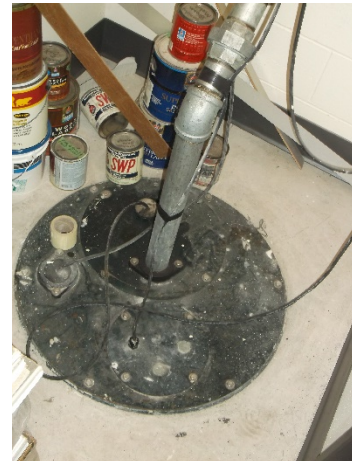
Elevator sump/pump
