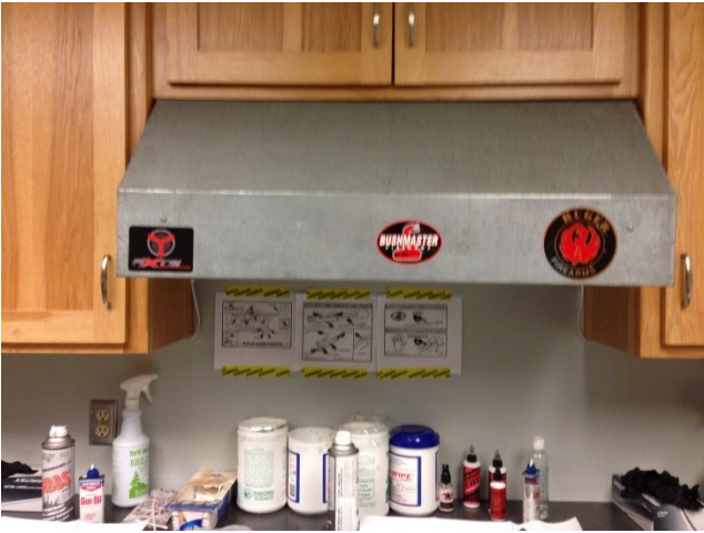
Firearm cleaning exhaust hood
