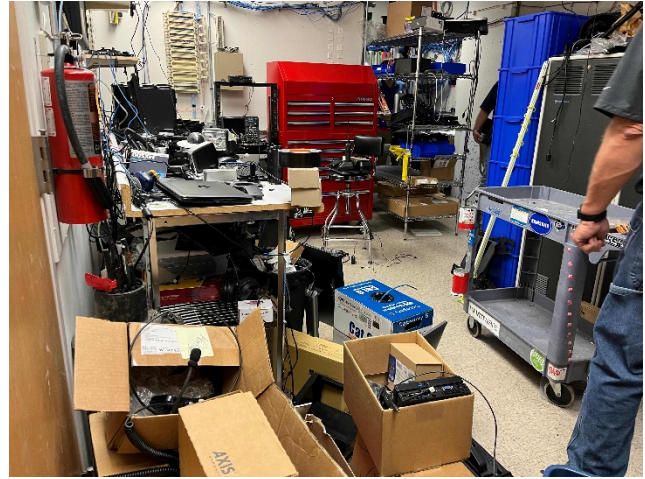
2nd floor IT room – improve egress route
