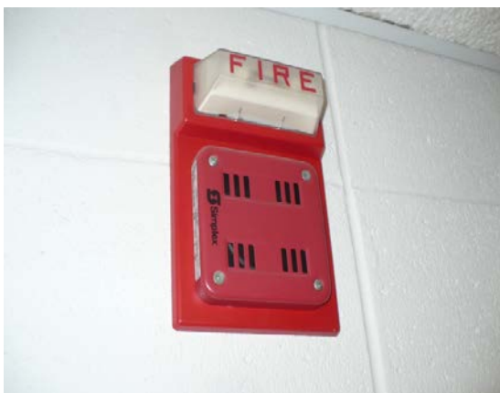
Fire alarm horn/strobe
