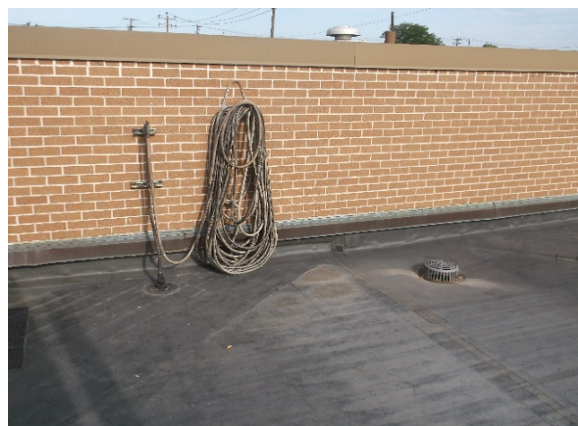
Sill faucet, roof drain
