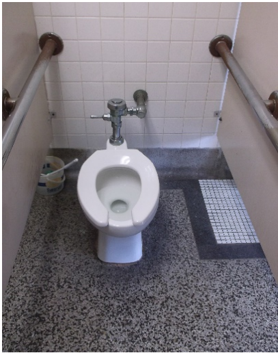
Water closet – men's
