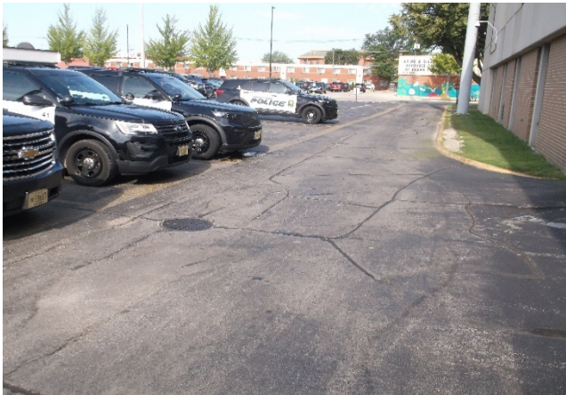
Parking Lot – South
