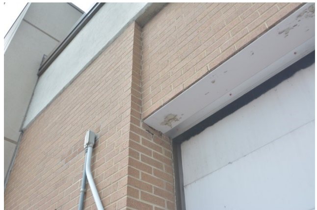
Lintels at garage door openings
