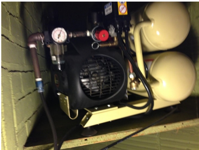
Temperature control air compressor
