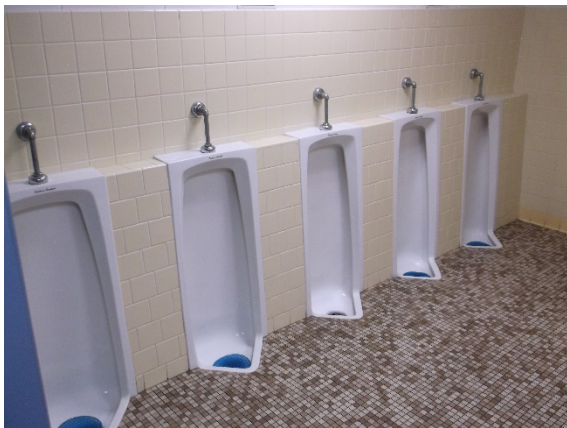
Men's toilet room – urinals
