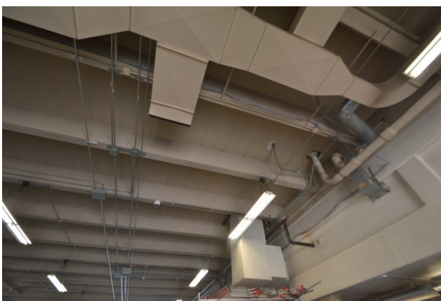
Roof structure at garage bay
