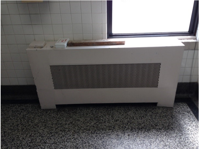
Radiation unit (typical)
