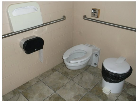
WC – ADA (typical per floor)
