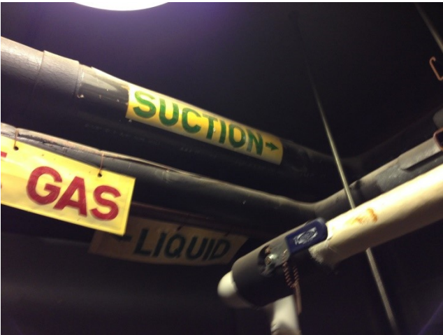
Good insulation (typical)
