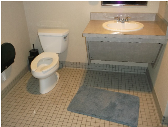
Water closet – judge's toilet room
