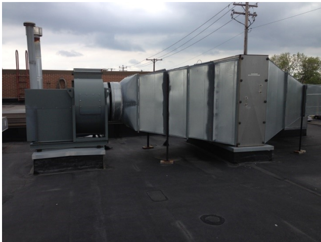
Firing range exhaust
