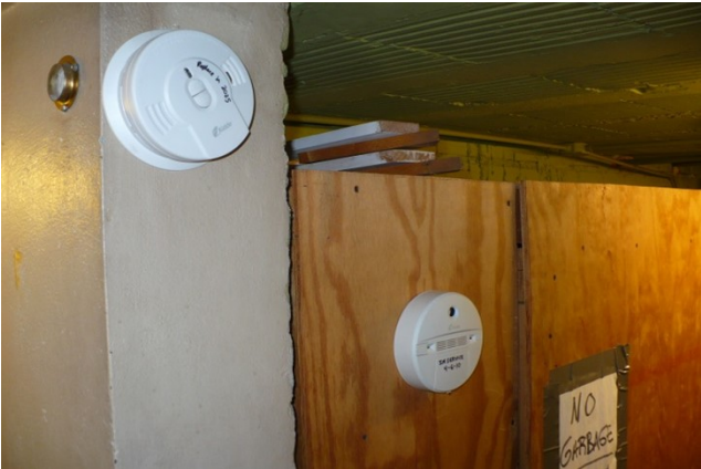
Stand-alone smoke & carbon monoxide detectors
