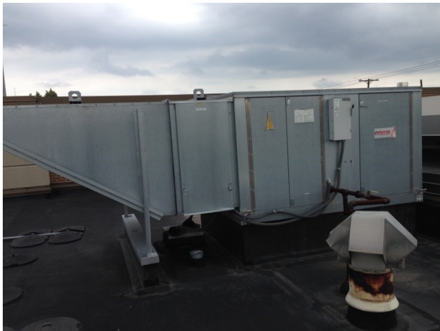
Firing range air unit
