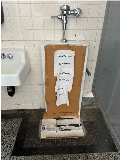
Remove unused fixture
