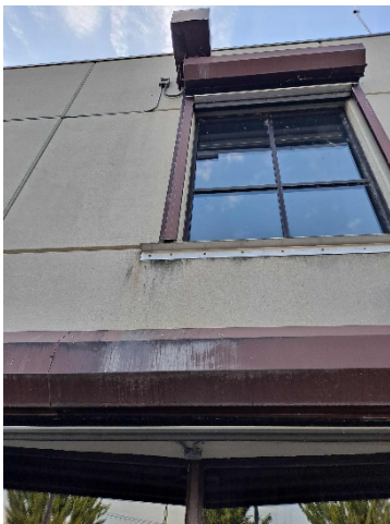
Window housing faded and rusting
