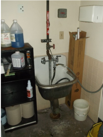
Inspector's test drain discharging in sink
