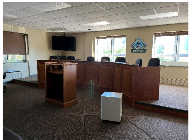
Committee room platform not accessible
