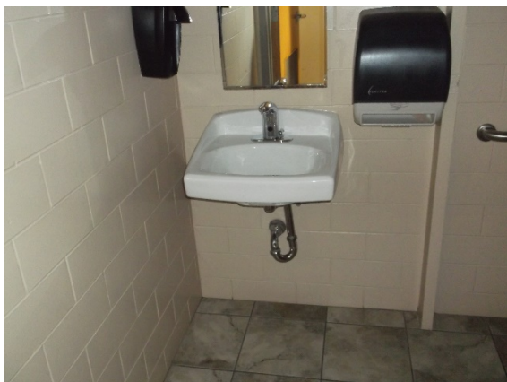
Lavatory – ADA (typical per floor)
