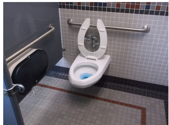
Water closet – 1 st floor public men's
