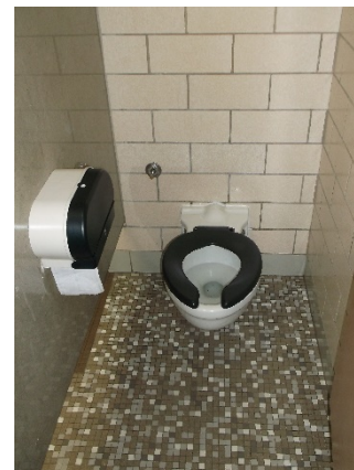
WC – public toilet room
