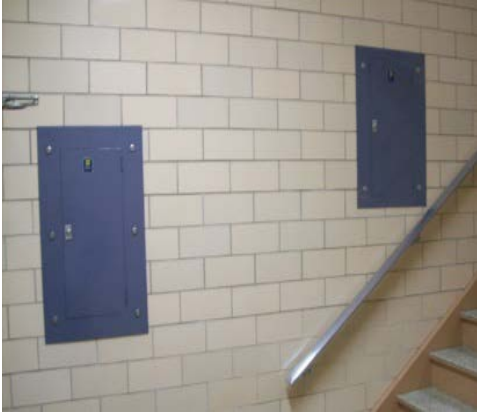
Panels in stairway
