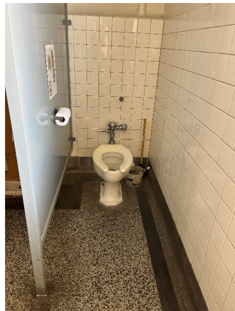
Potential area for accessible toilet
