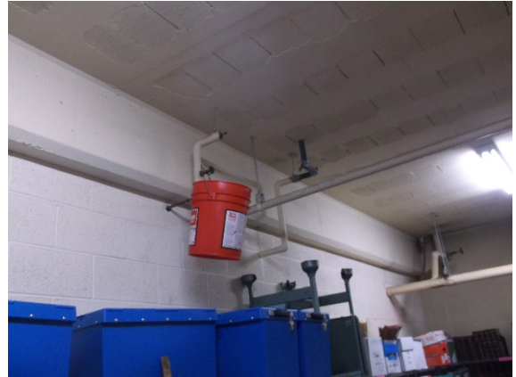
Leaking valve(s)
