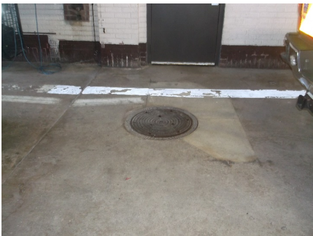
Garage catch basin
