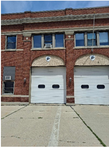
Exterior brick in good condition
