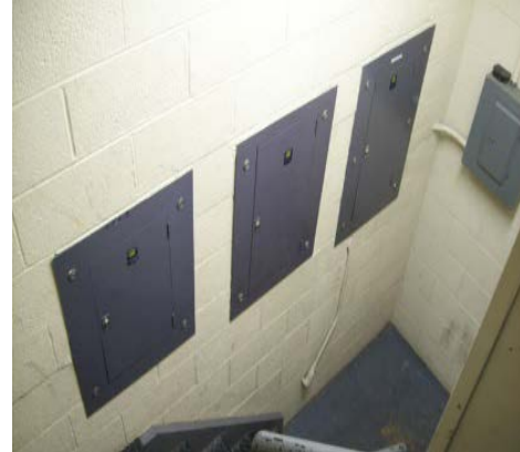
Panels in stairwell to penthouse
