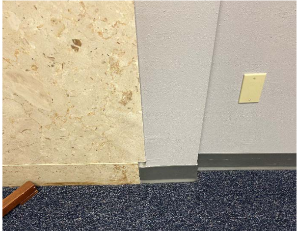
Fill gap in wall
