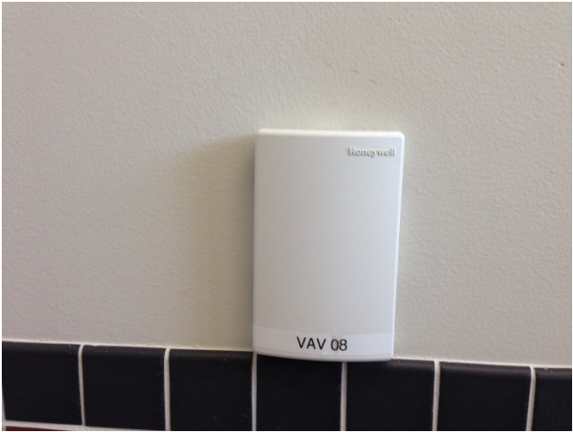
Low voltage thermostat
