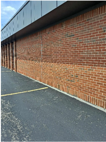
Exterior brick in good condition
