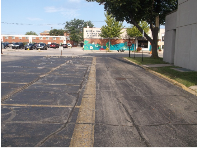
Parking Lot – South
