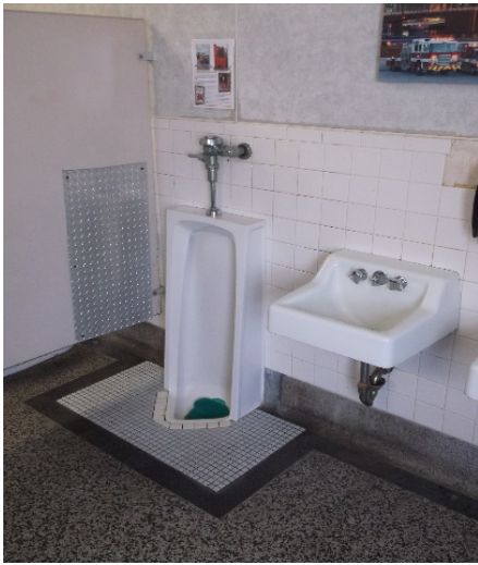
Urinal & lavatory – men's
