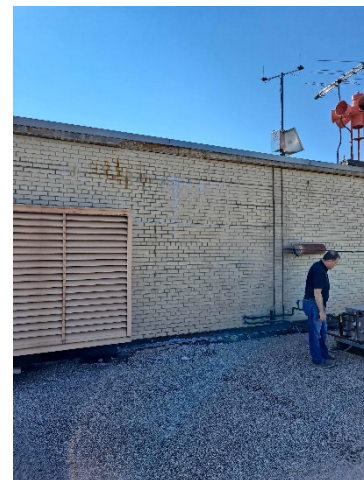
Mechanical penthouse - tuck pointing
