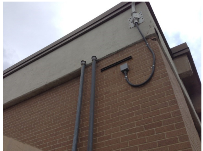
Fuel tank vents
