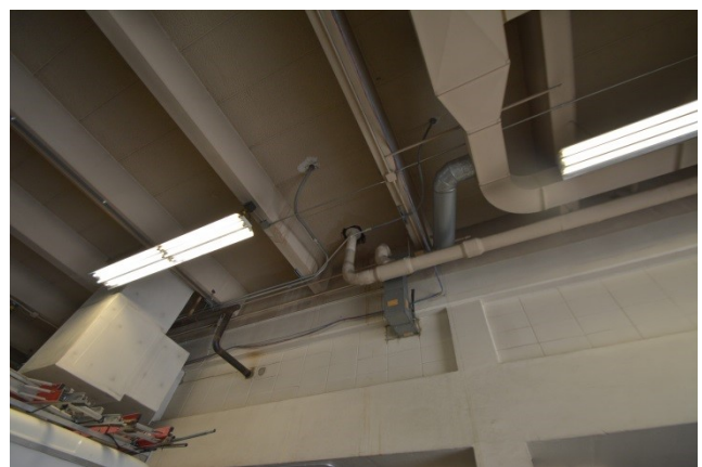
Roof bearing at office/garage supporting wall
