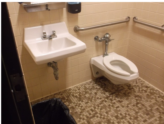
Staff toilet room – 1 st floor
