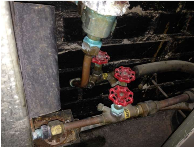
Typical induction unit piping
