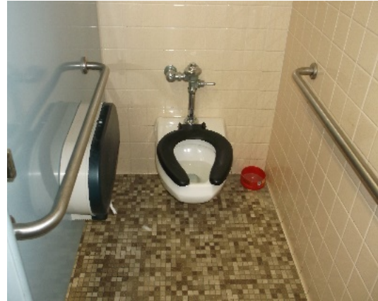
Water closet – basement men's
