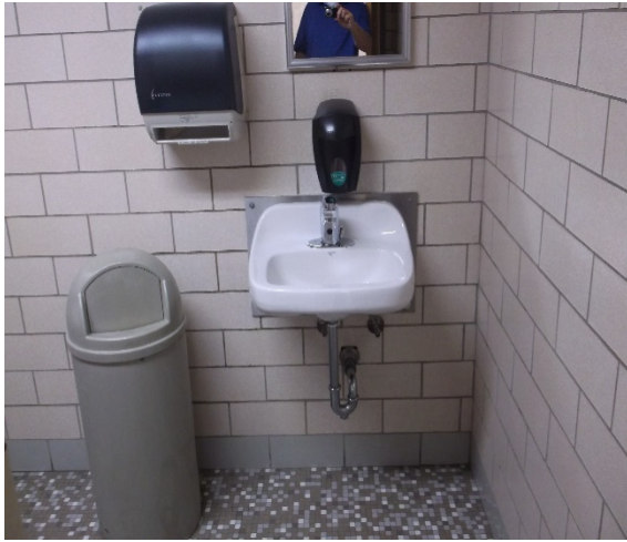
Lavatory – public toilet room
