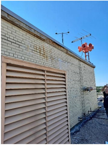
Penthouse pre-cast coping replacement
