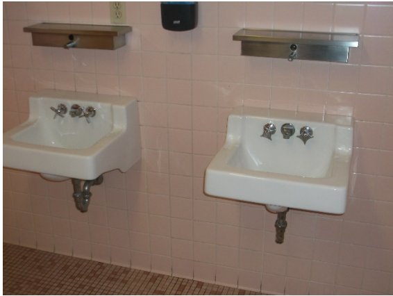
Lavatories – basement women's
