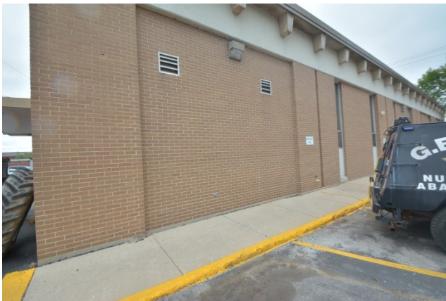
Concrete roof purlins at garage
