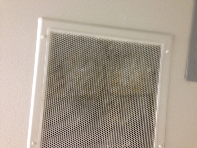
Old grille (plugged)
