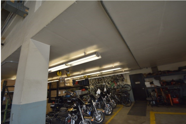
2 nd floor plan structure as seen from garage
