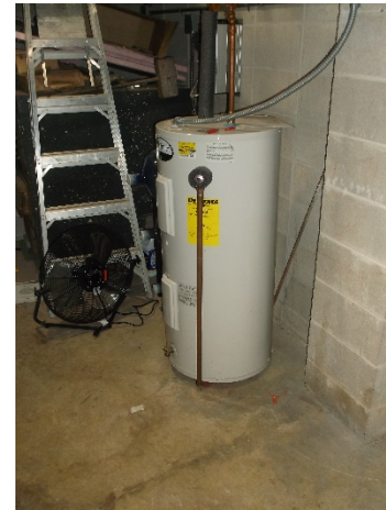
Electric water heater
