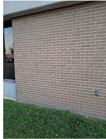
Brick in good condition
