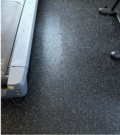
Gap in rubber floor tile
