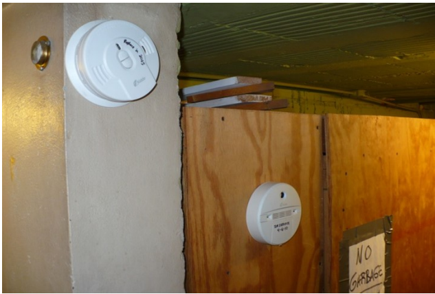
Stand-alone smoke & carbon monoxide detectors
