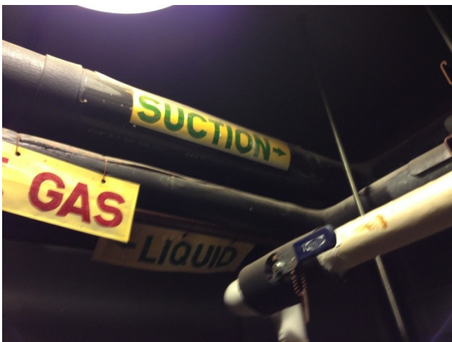
Good insulation (typical)
