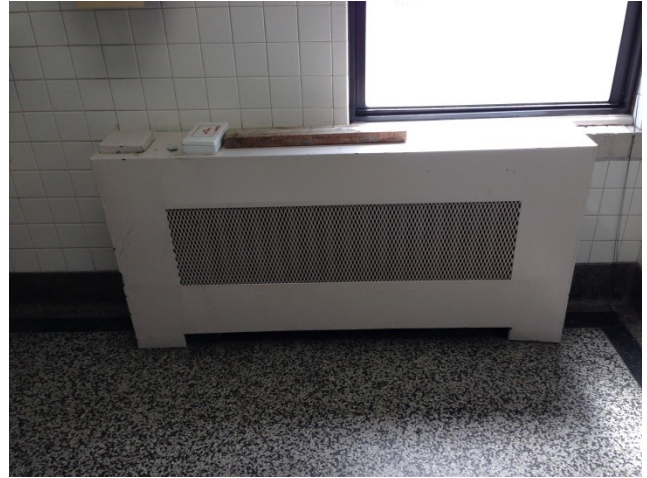
Radiation unit (typical)
