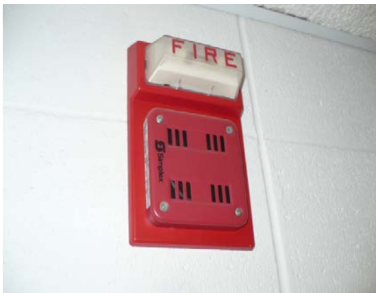
Fire alarm horn/strobe
