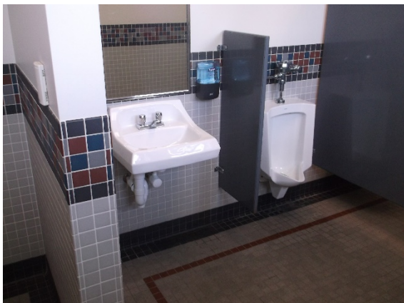
Lavatories – 1 st floor public men's
