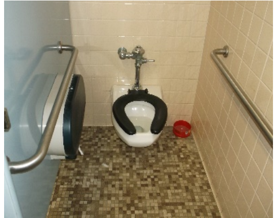
Water closet – basement men's
