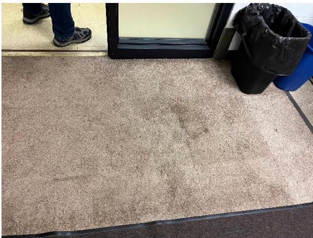
Worn, stained cut-pile carpet
