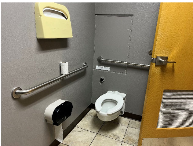
3 rd floor: grab bar mounted on panel
