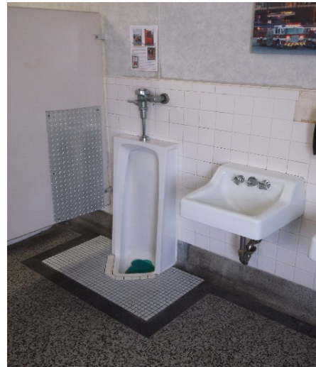
Urinal & lavatory – men's
