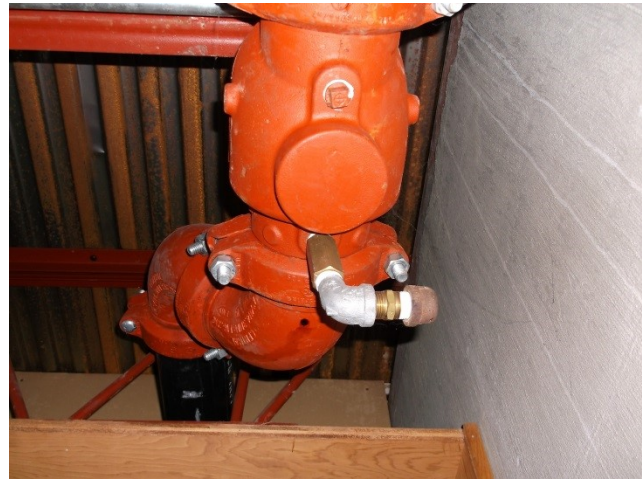
Automatic ball drip capped
