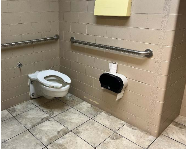
Peeling paint from glazed block
