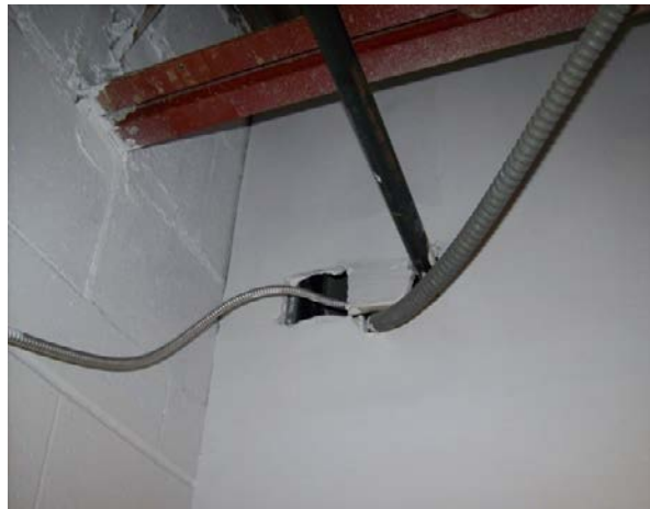
Opening through wall common with stairway
