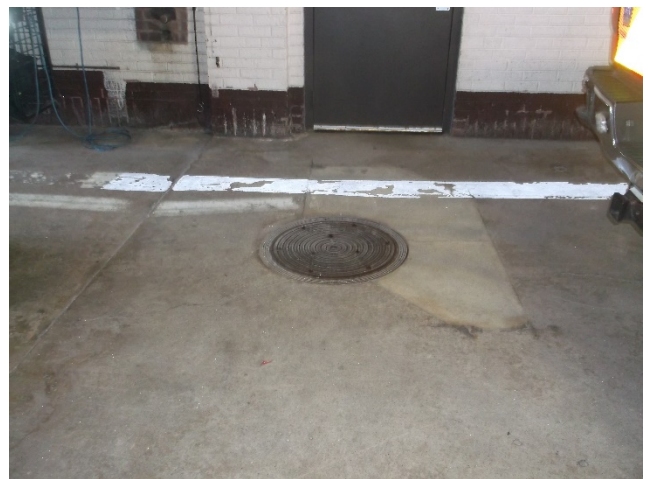
Garage catch basin
