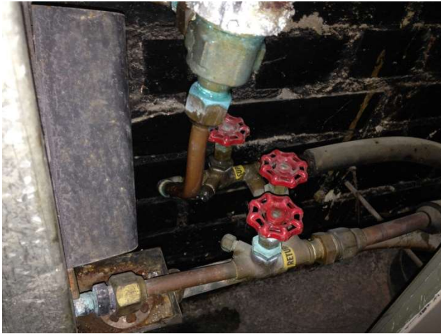
Typical induction unit piping
