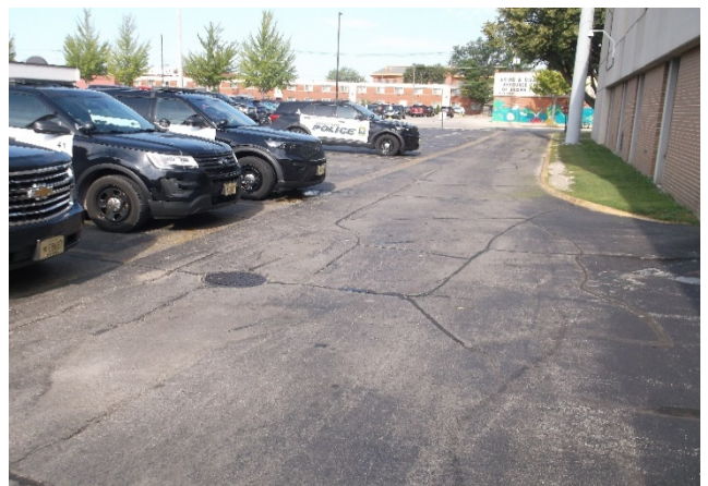
Parking Lot – South
