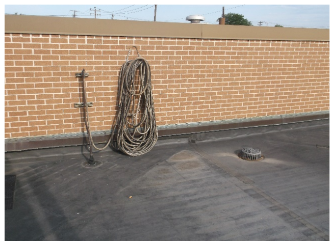
Sill faucet, roof drain
