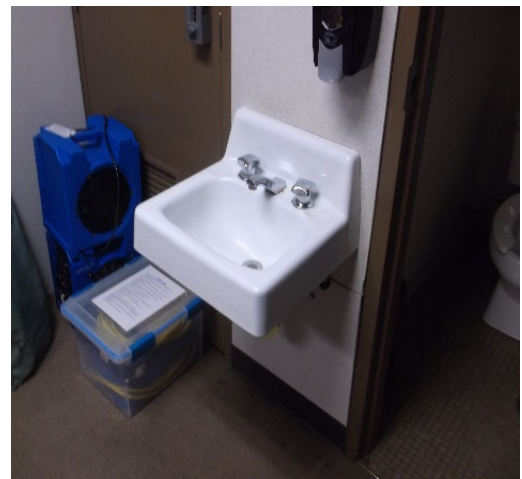
Lavatory – outside unisex toilet room
