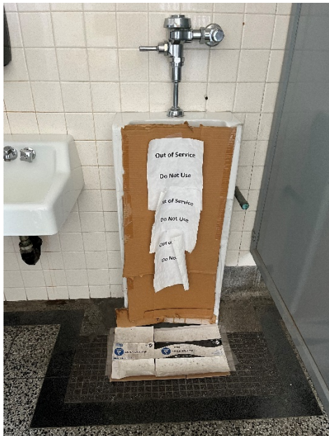
Remove unused fixture
