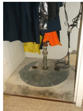
Elevator sump/pump
