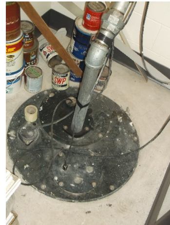
Elevator sump/pump
