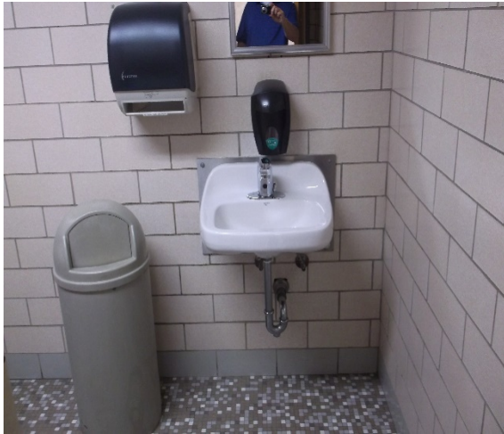
Lavatory – public toilet room
