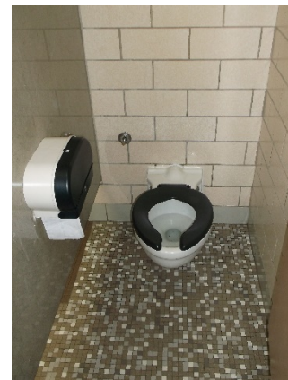
WC – public toilet room
