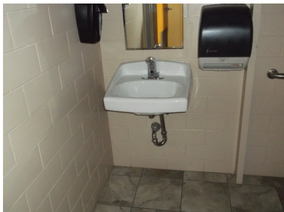
Lavatory – ADA (typical per floor)
