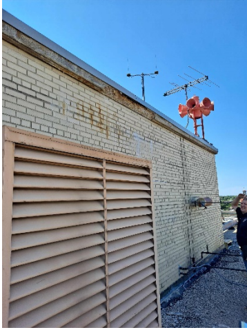
Penthouse pre-cast coping replacement
