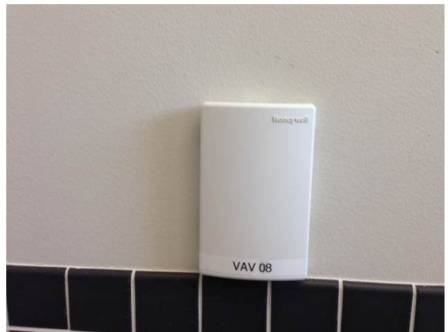
Low voltage thermostat
