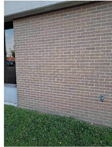
Brick in good condition
