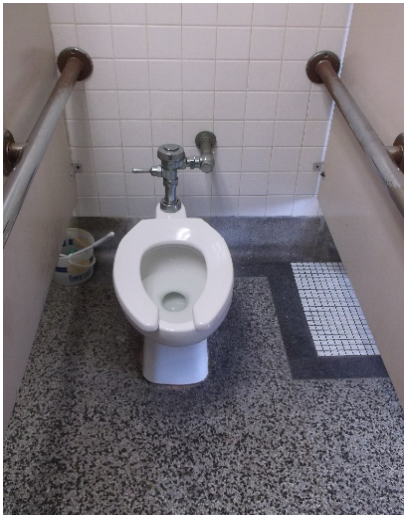
Water closet – men's
