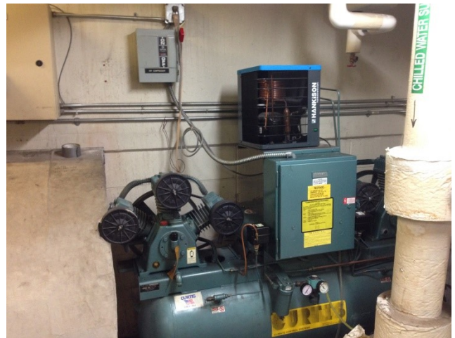
Temperature control air compressor
