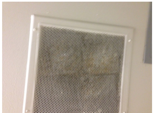
Old grille (plugged)
