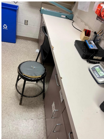
Plastic laminate casework condition
