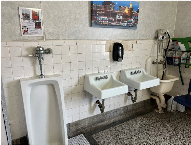
Recommend lever faucet handles
