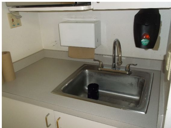
Break room sink
