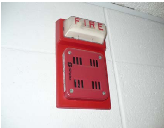
Fire alarm horn/strobe
