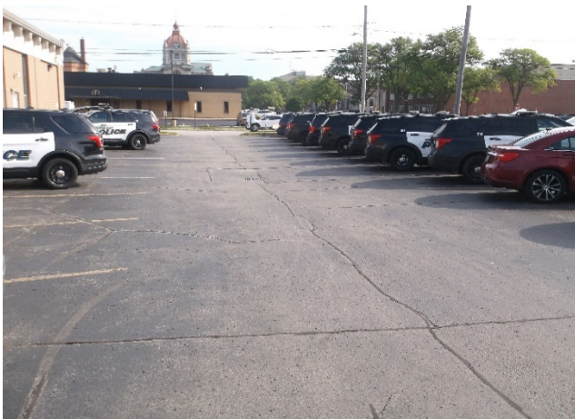
Parking Lot – East
