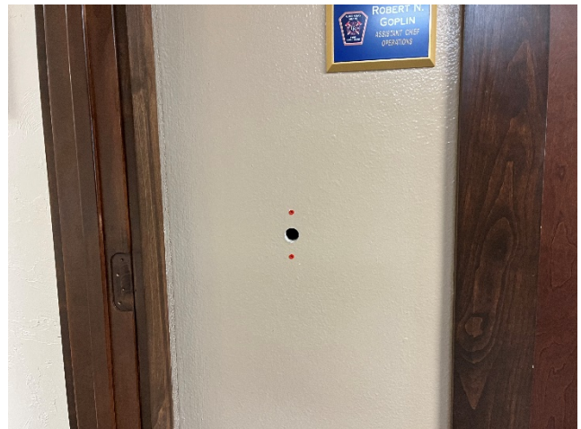
Patch hole in wall
