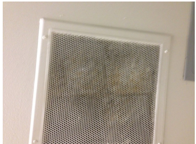
Old grille (plugged)
