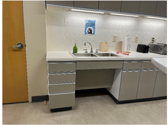
Sink with front-approach accessibility
