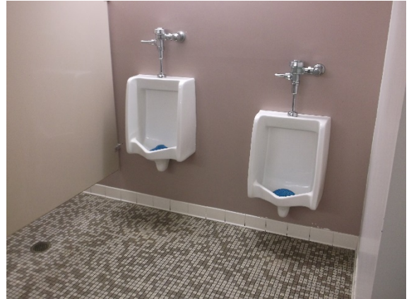
Men's toilet room
