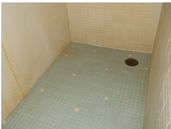
Men's shower room floor drain
