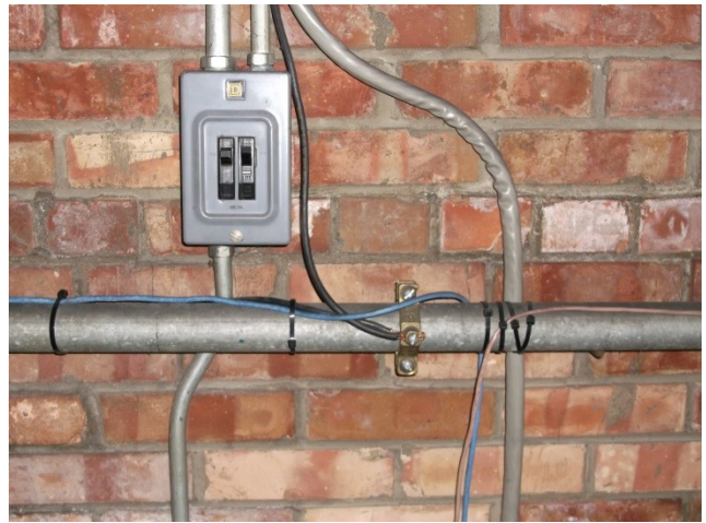
Cable attached to standpipe
