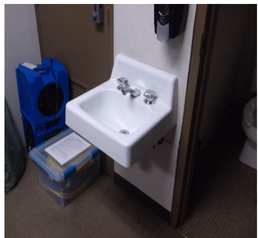
Lavatory – outside unisex toilet room
