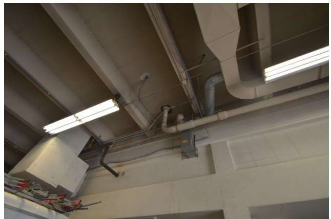
Roof bearing at office/garage supporting wall
