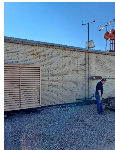
Mechanical penthouse - tuck pointing
