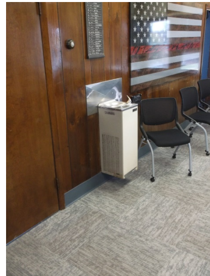
Electric water cooler- meeting room
