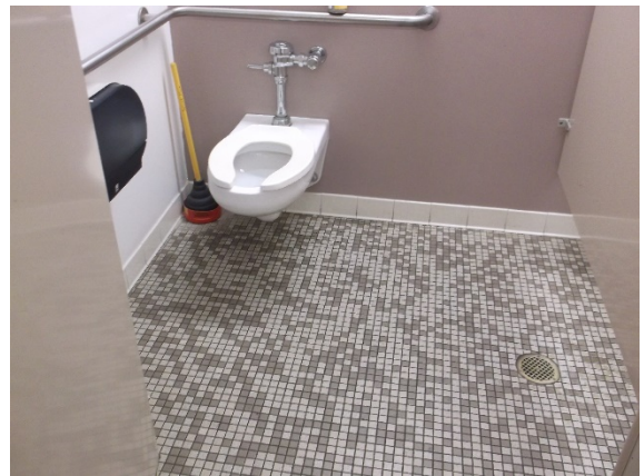
Men's toilet room
