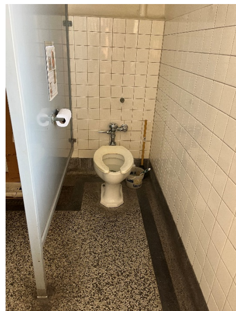
Potential area for accessible toilet
