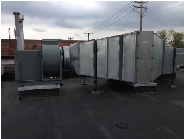
Firing range exhaust
