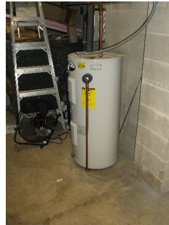
Electric water heater
