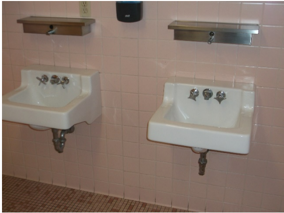
Lavatories – basement women's
