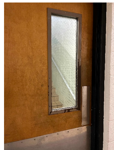
Chipped paint at lite and damaged wood finish
