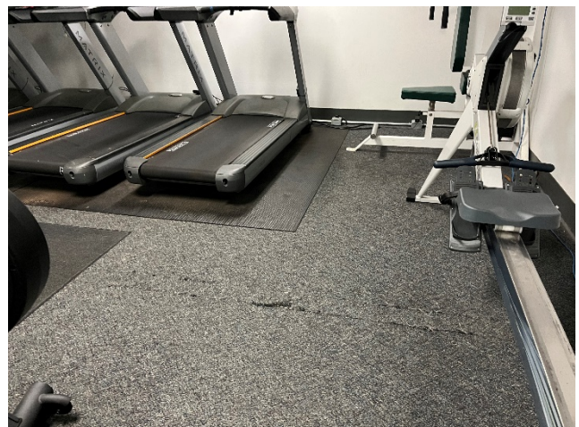
Ripped carpet at cardio room
