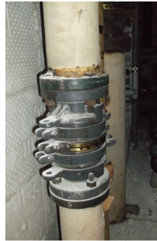
Expansion joint (4th floor) toilet chase
