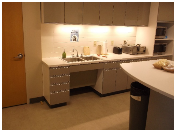
Kitchen sink – 6 th floor
