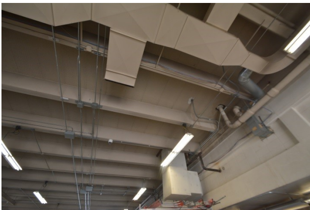
Roof structure at garage bay
