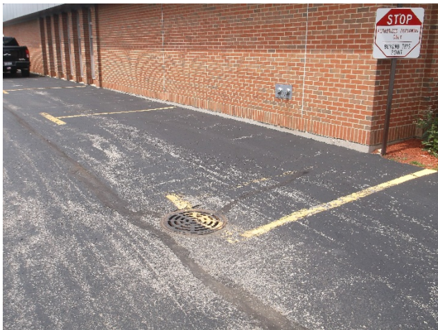
Parking lot- catch basin
