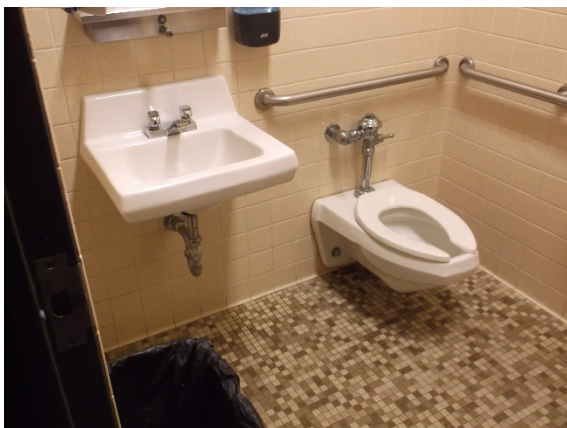
Staff toilet room – 1 st floor
