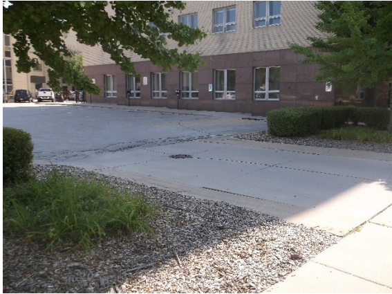
Parking lot - north
