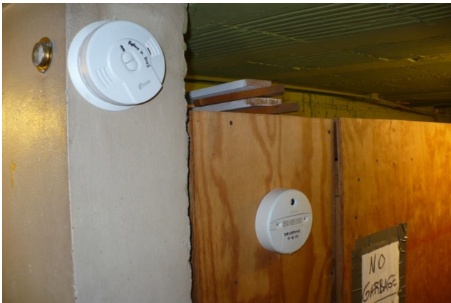
Stand-alone smoke & carbon monoxide detectors
