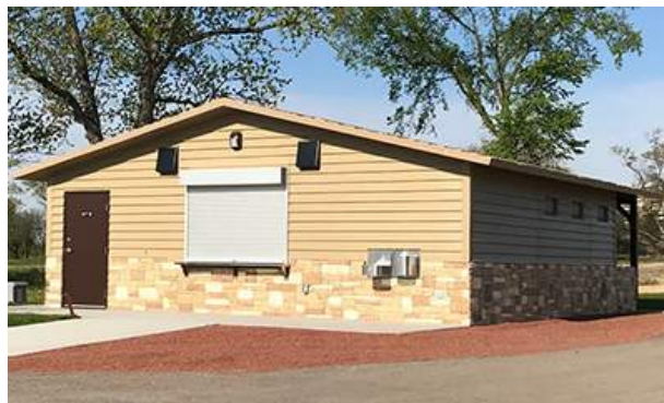
Precast Restroom Structure
