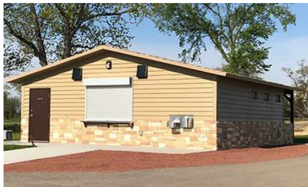
Precast Restroom Structure
