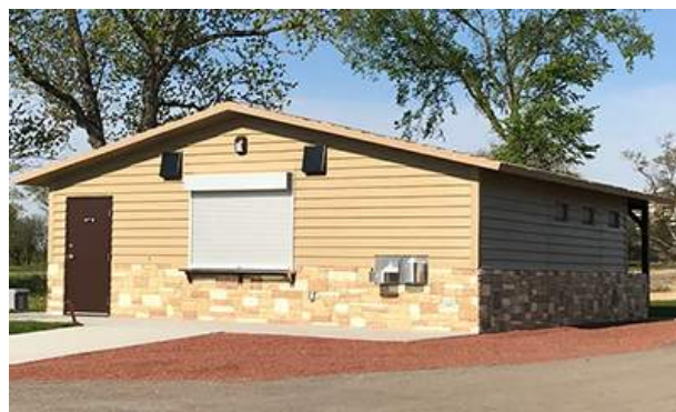
Precast Restroom Structure
