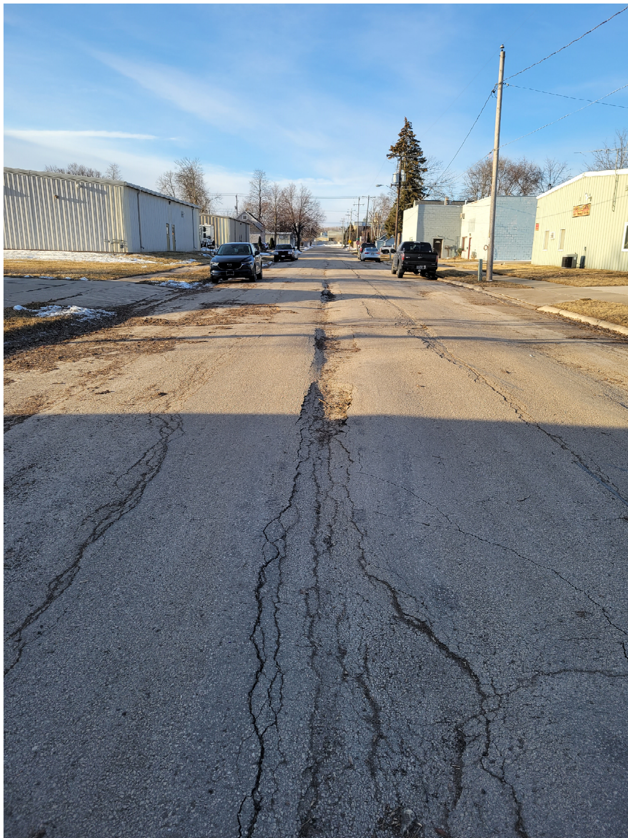
3/10/22 Existing Condition – Looking South towards Ninth Street
