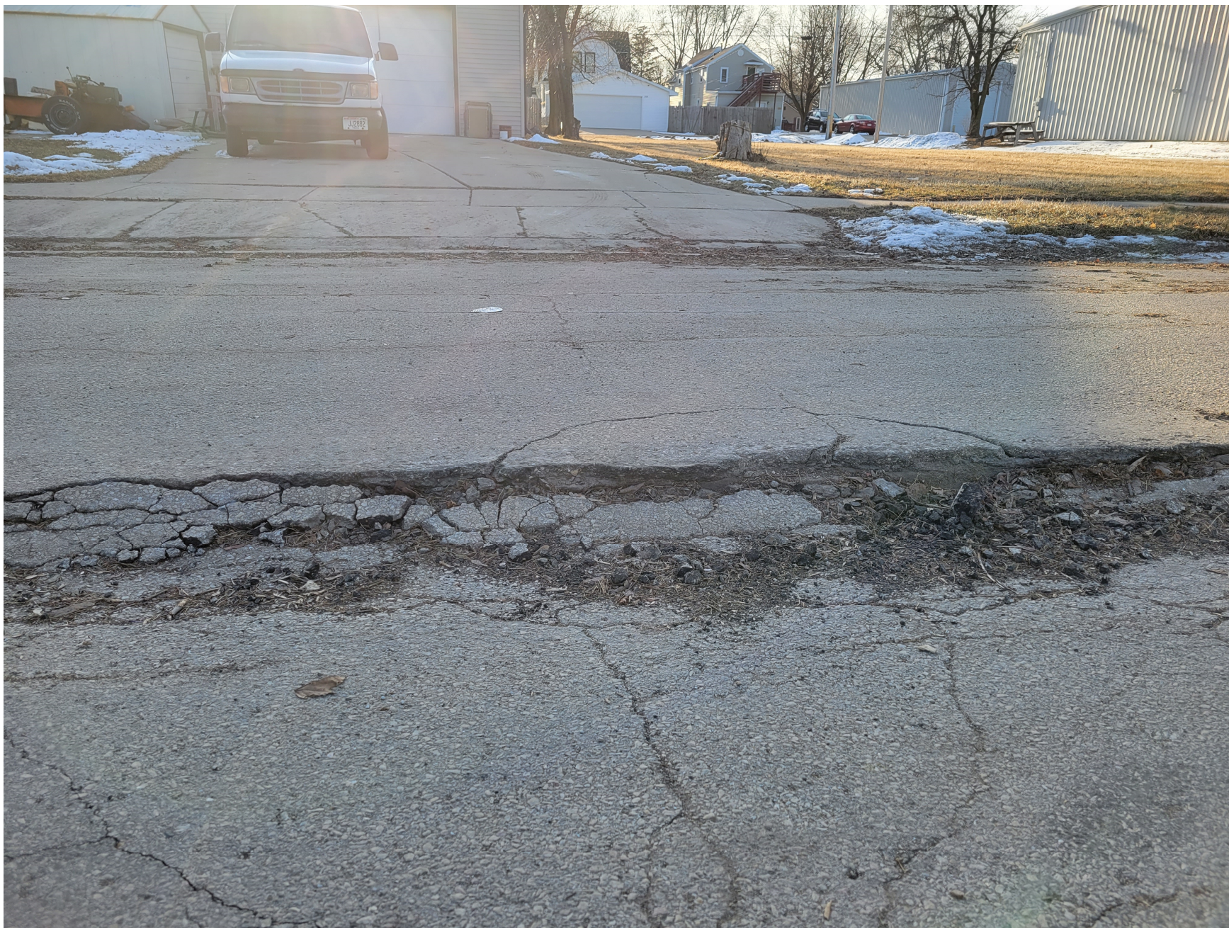
3/10/22 Existing Condition – Looking West
