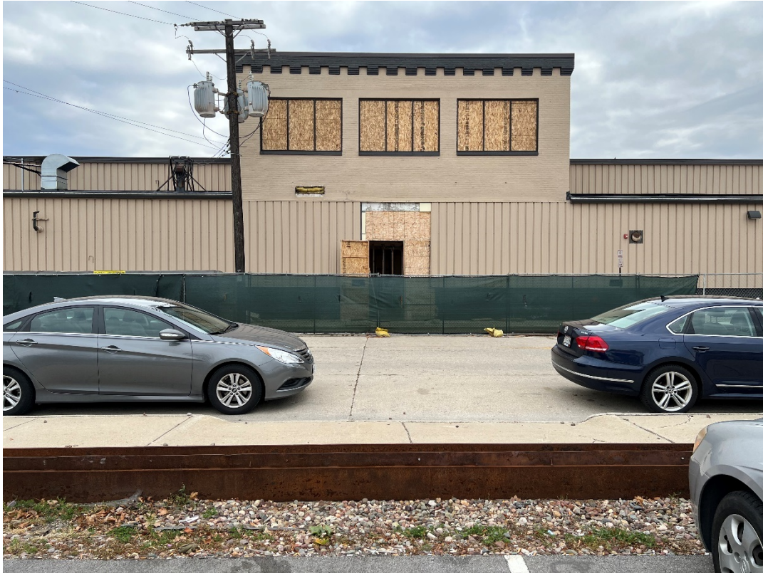
Figure 2 – North Driveway (Inactive), Crown & Common, Looking East at the Pomp's Tire Building
