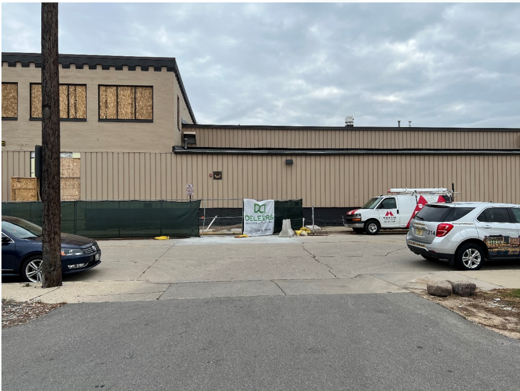
Figure 3 – South Driveway (Active), Crown & Common, Looking East at the Pomp's Tire Building
