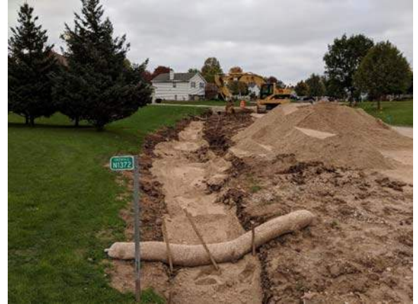
STREET RAIN GARDEN
