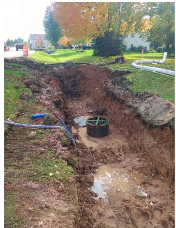
DOUBLE RING INFILTRMETER TESTING
