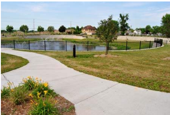
Trail, retaining wall, railing, bollard lights, and landscape beds
