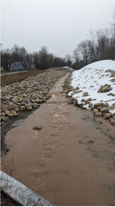
Brown County Bay Beach Lane and Eagles Nest Boat Launch Drainage Project
