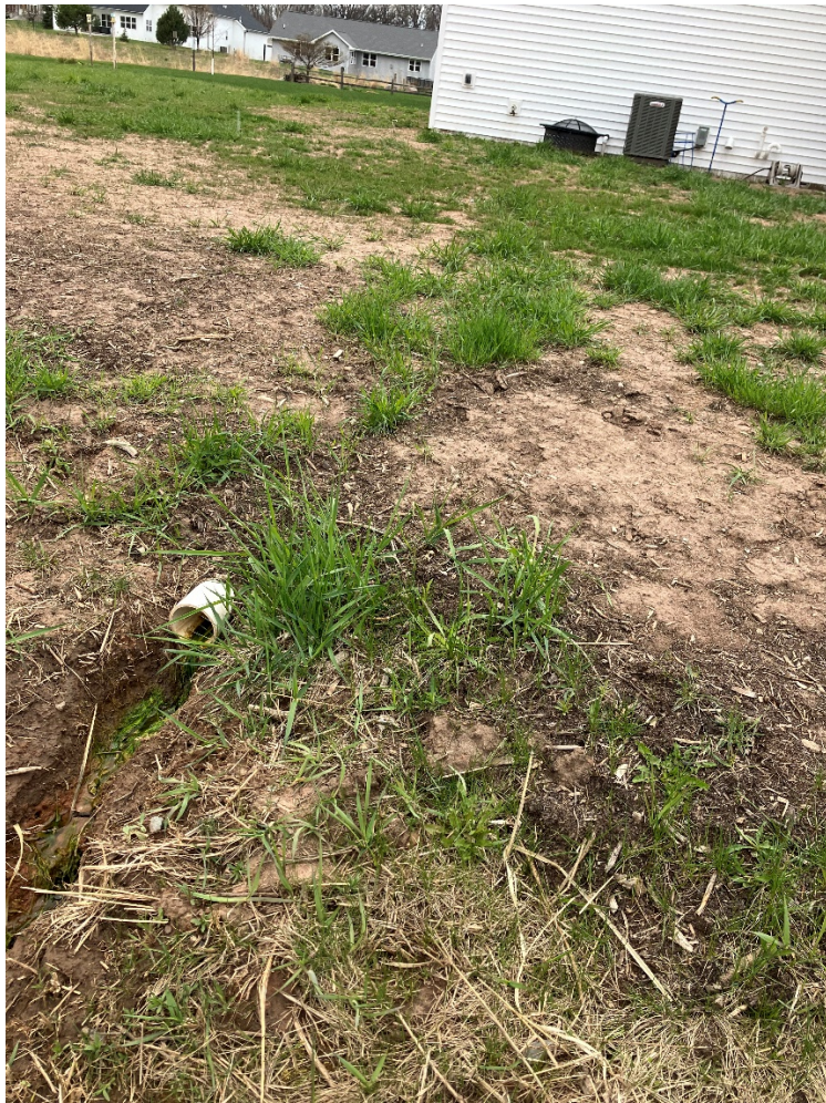
Current pipe discharging to City Owned Storm Water Drainage
