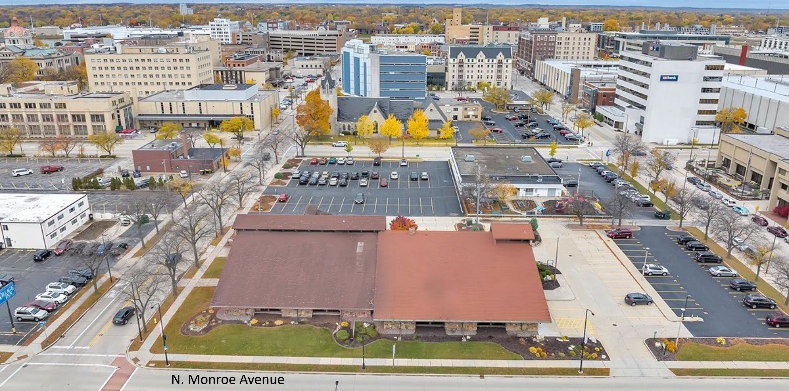
201 N. Monroe, Green Bay, Wisconsin View from N Monroe Avenue
