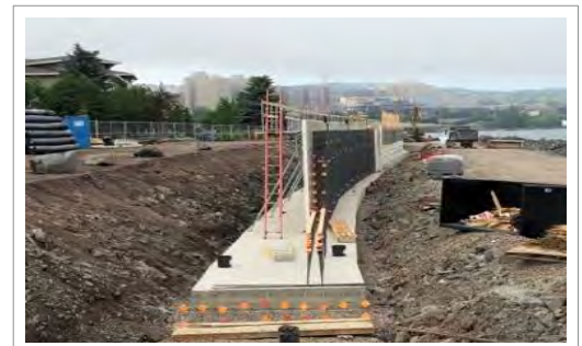
Concrete Wall Construction
