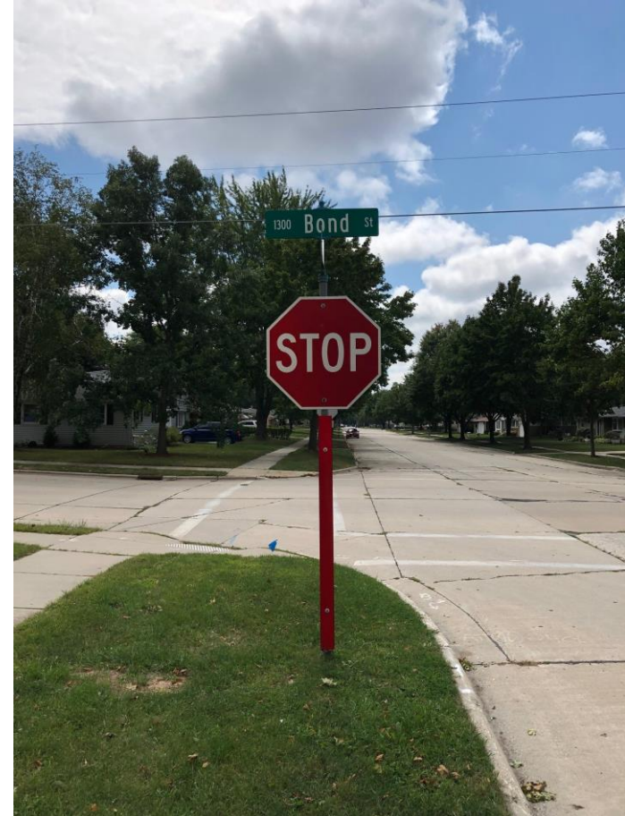
Example: Added Brite Side to existing sign support post
