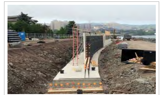
Concrete Wall Construction
