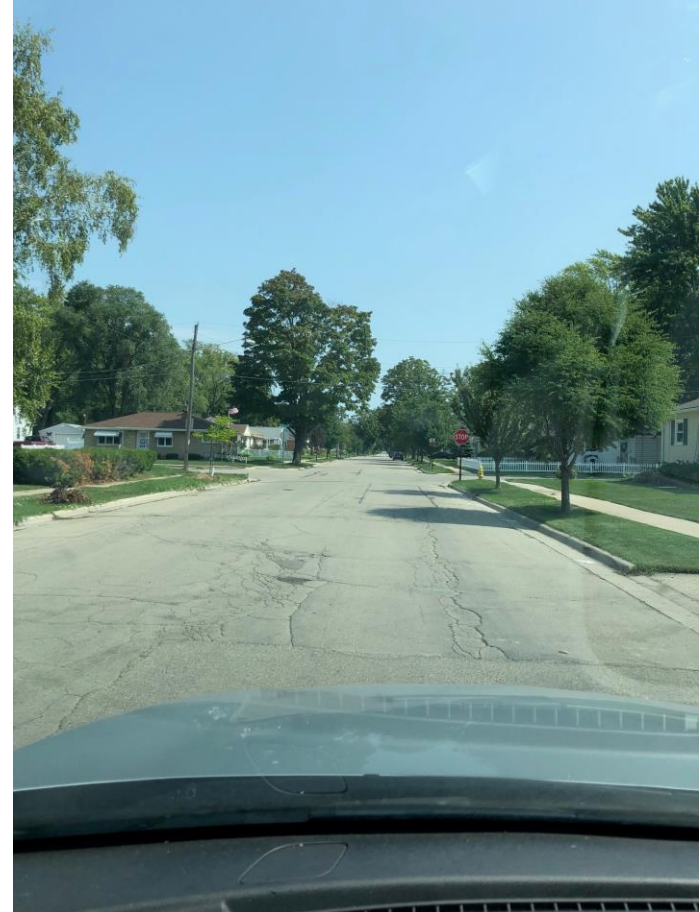
Eastbound Bond at Wilson Stop Sign Stop. City recently moved Stop closure to back of curb to make it more visible. Crab Apple trees could be trimmed or removed. We could add STOP ADVANCE and add Brite side to both sign supports.
