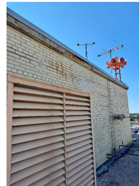
Penthouse pre-cast coping replacement
