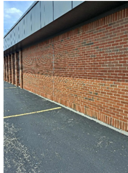
Exterior brick in good condition
