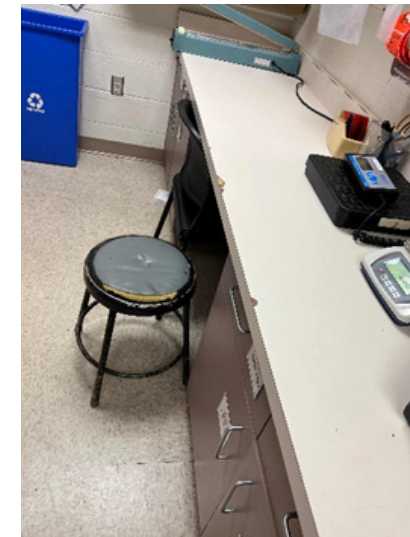
Plastic laminate casework condition
