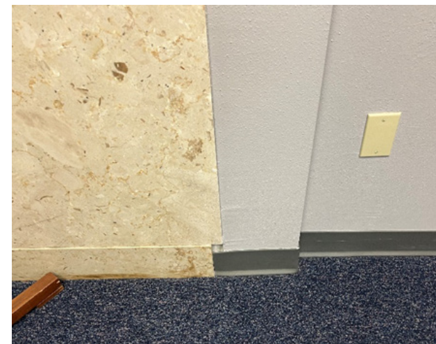
Fill gap in wall
