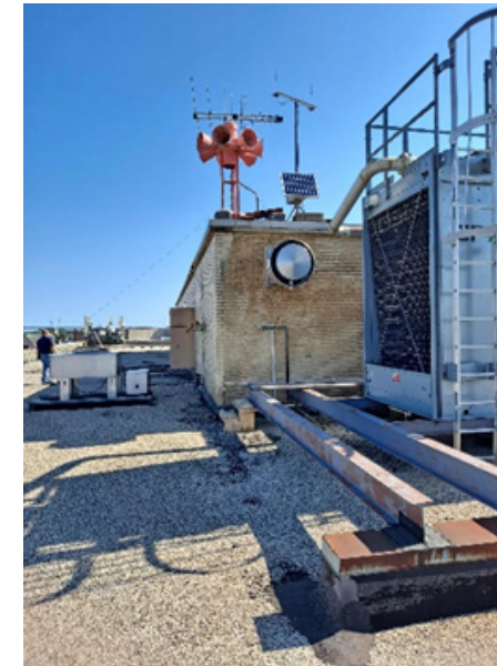
Existing roof - replace
