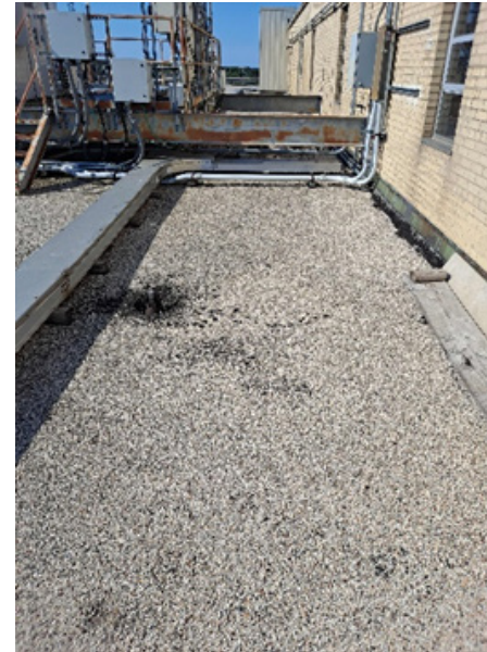
Existing roof - replace
