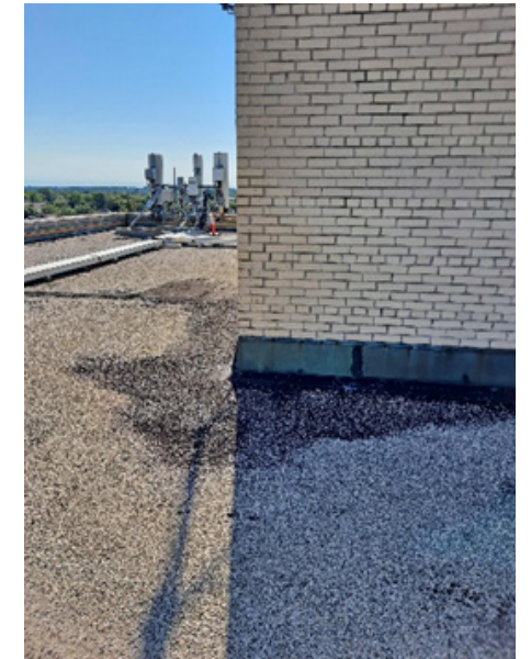
Mechanical penthouse - tuck pointing
