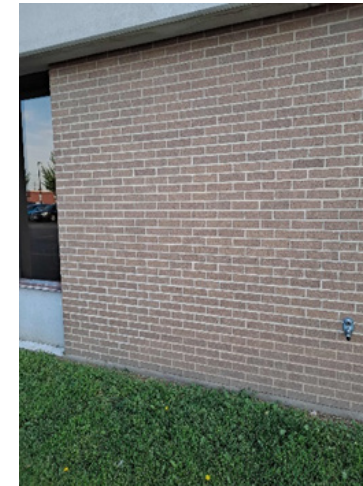
Brick in good condition
