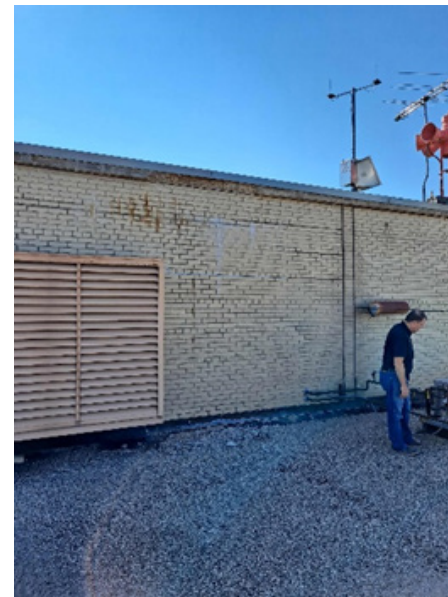
Mechanical penthouse - tuck pointing
