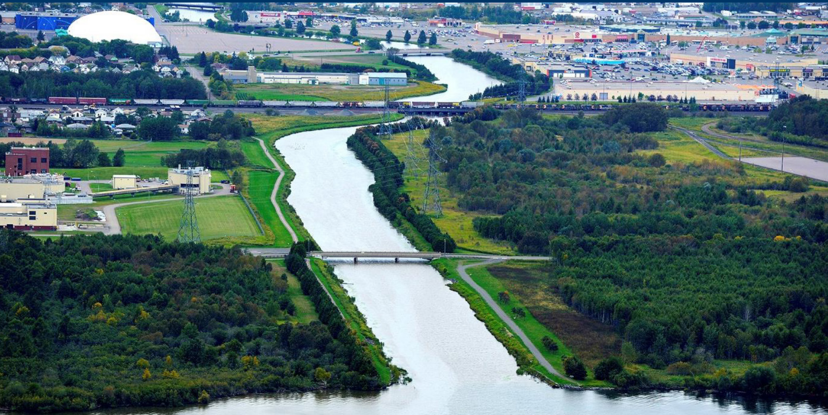
Neebing-McIntyre Floodway looking upstream from Lake Superior. City of Thunder Bay, ON. (LRCA n.d.)
