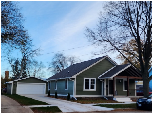
331 S Irwin Ave Bridges Construction/NeighborWorks
