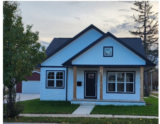
1200 Doty Street LeMense Construction
