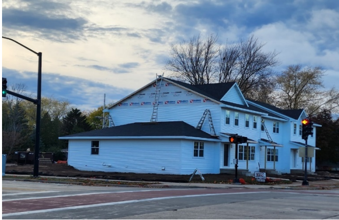
Walnut/Baird Street JAS House Estimated Completion 12/23
