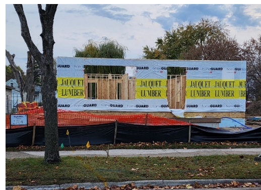
1164 Day Street Bridges Construction/NeighborWorks
