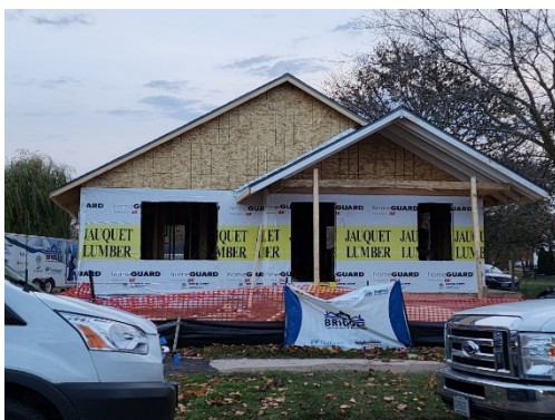
1162 Day Street Bridges Construction/NeighborWorks
