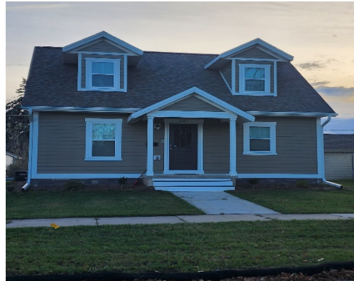
421 4 th Street Bridges Construction/NeighborWorks
